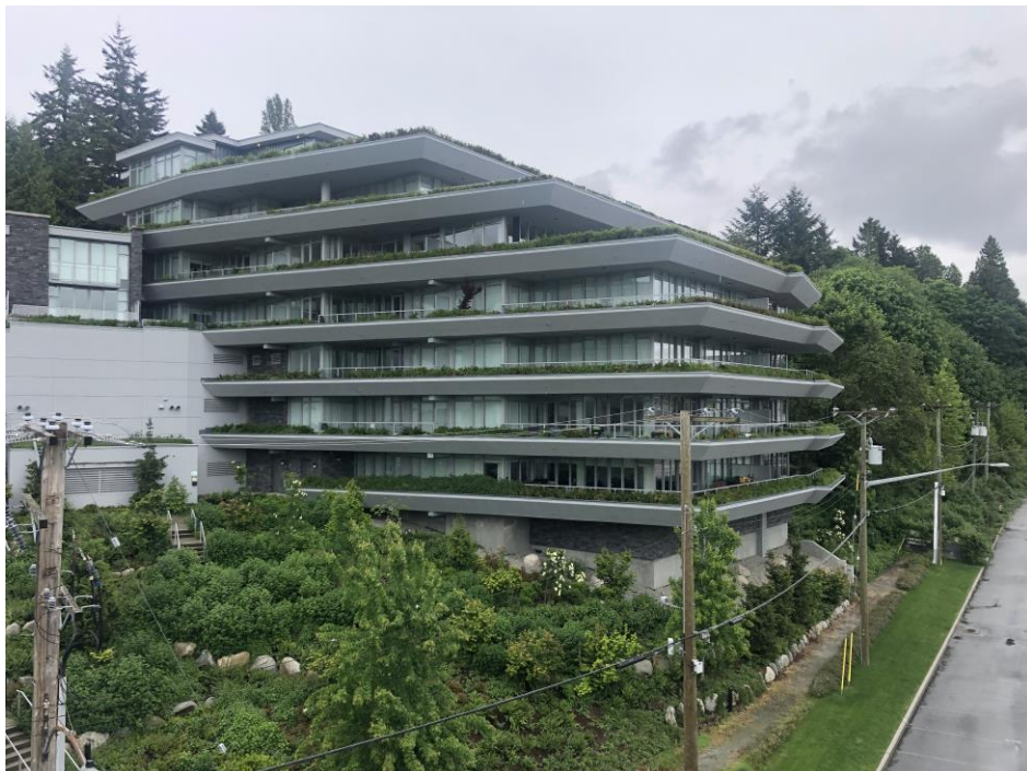
Figure 6a: Resident mews at Lot 7 (southern path shown lower right)
