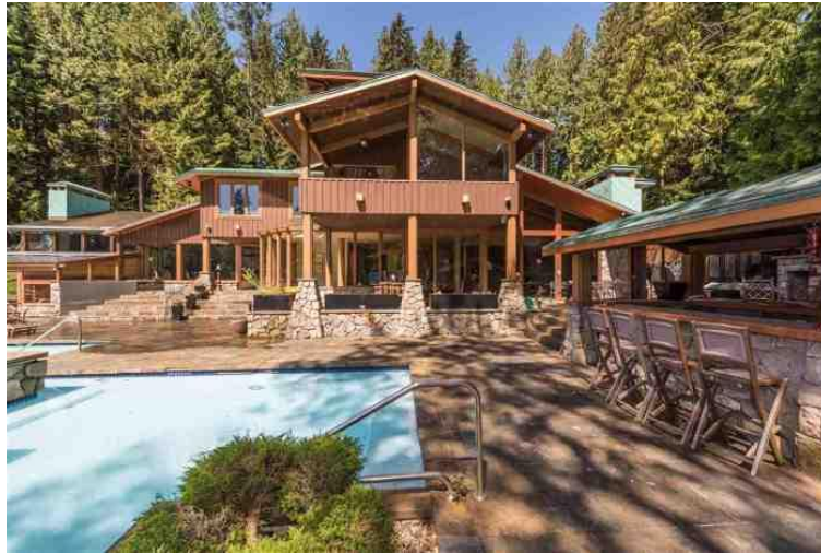
Figure 3: Recent photo of the east elevation (rear) of the Hall Residence
