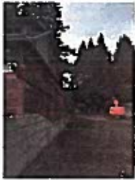
109 WEST NEIGHBOR LOOKING NORTH
