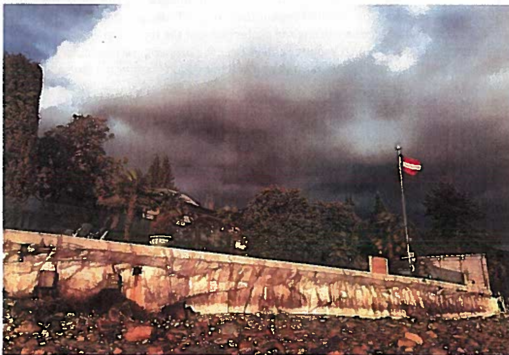
Figure 5. Neighbouring property east of the study site.
