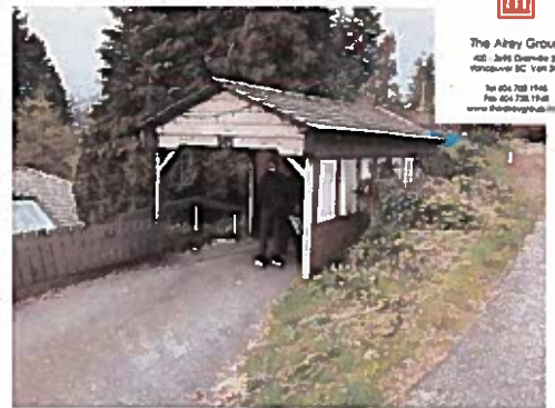
VIEW OF EXISTING CARPORT FROM LANE
