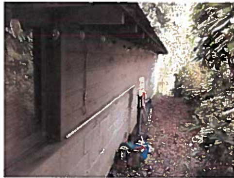
VIEW LOOKING NORTH ALONG EAST ELEVATION
