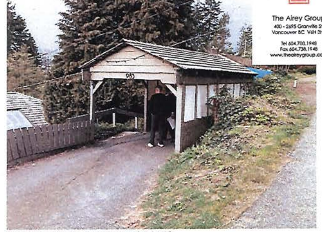
VIEW OF EXISTING CARPORT FROM LANE
