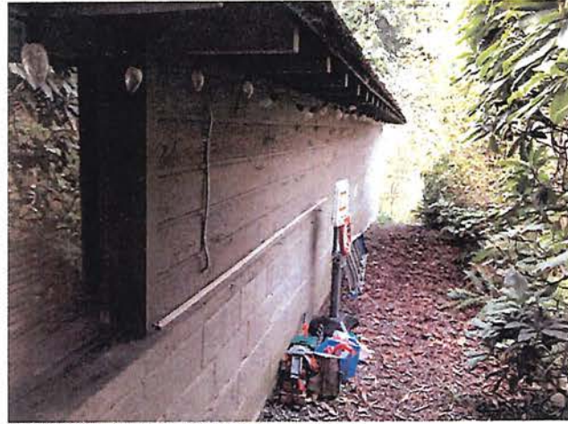
VIEW LOOKING NORTH ALONG EAST ELEVATION
