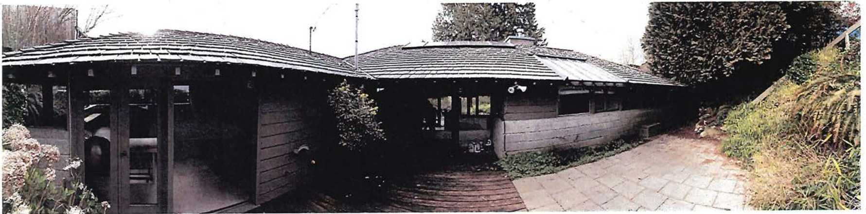
PANORAMIC VIEW OF NORTH ELEVATION
