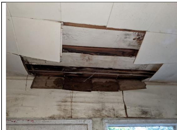
Photo 5: Exposed ceiling strapping on the upper floor.
