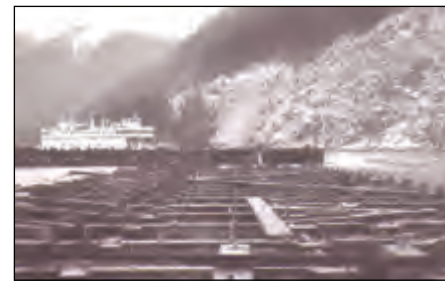
Installation of floating breakwater c. 1958
