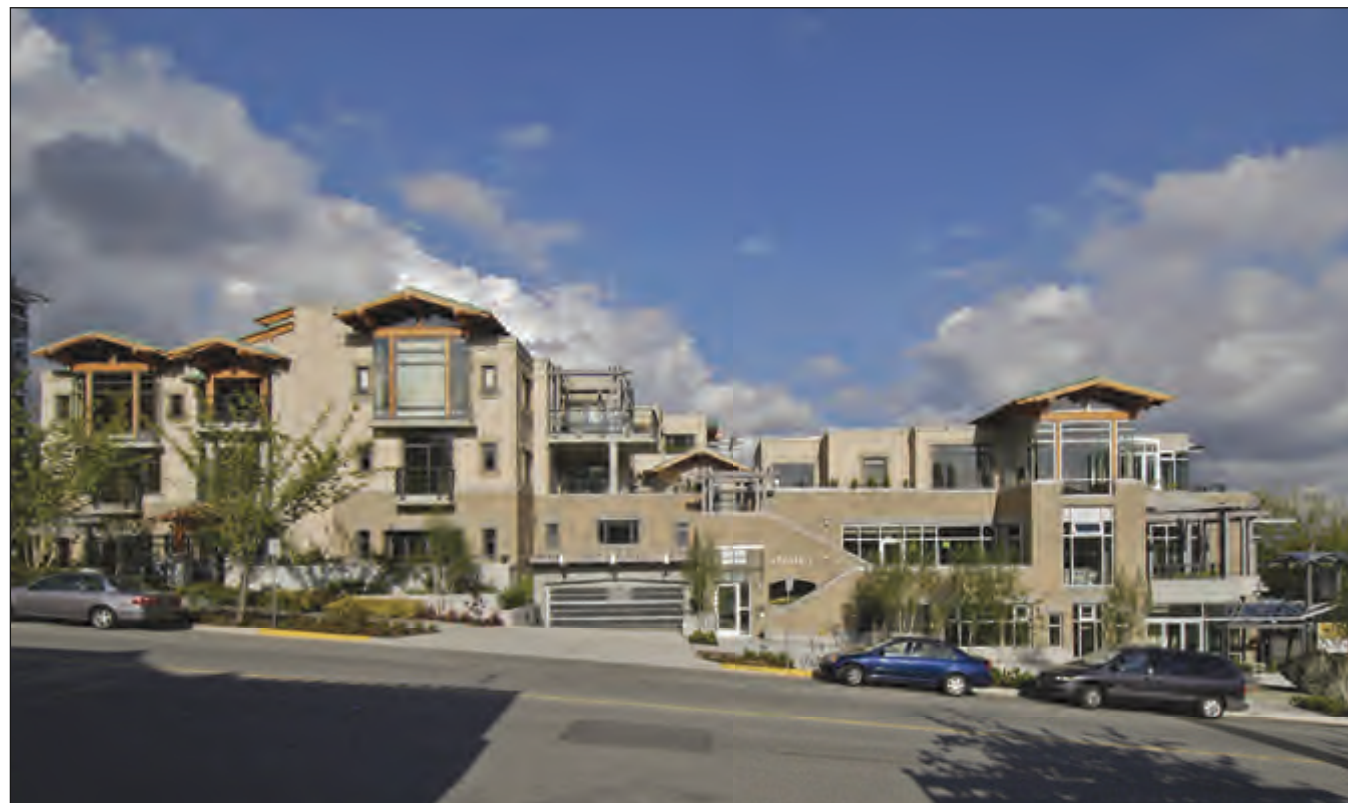
<< Riverway Golf Clubhouse Burnaby, BC by Merrick Architecture 2012
