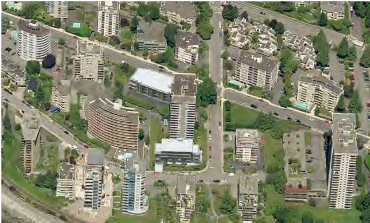
South Bird's Eye View - Bellevue & Argyle Buildings
