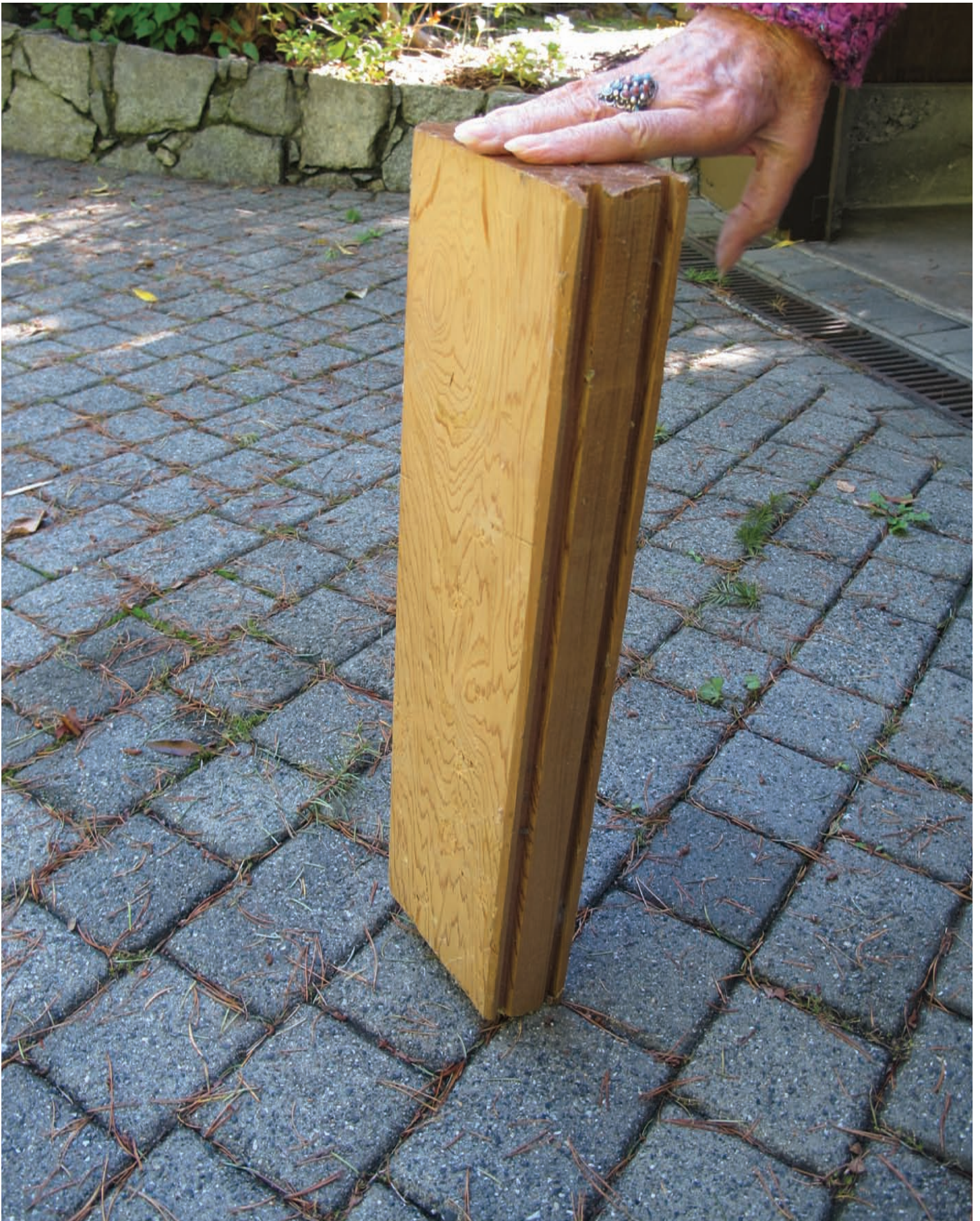
Tongue-and-groove ceiling panel: 10 centimetre thickness
