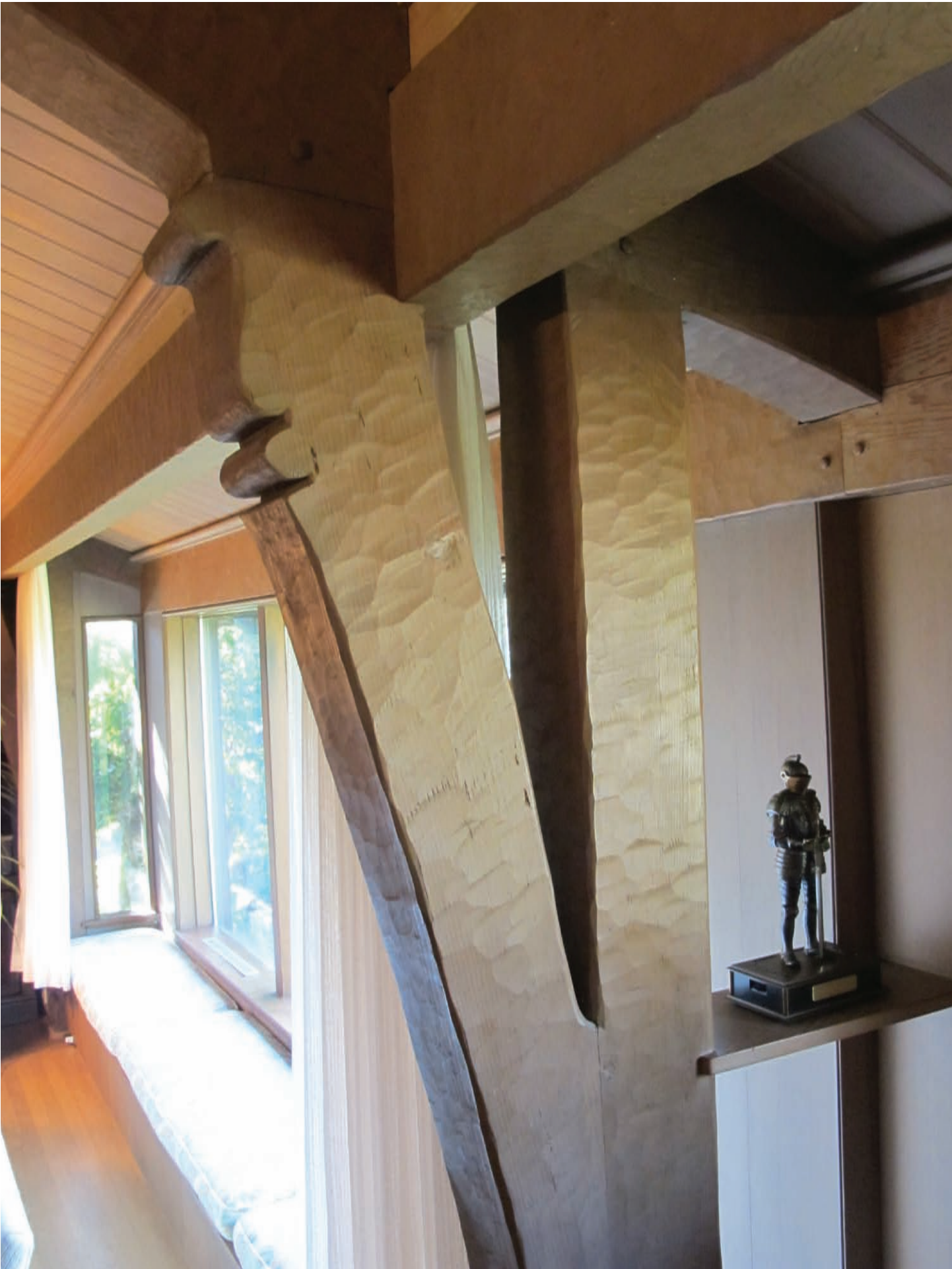
Hand adzed wooden post detail
