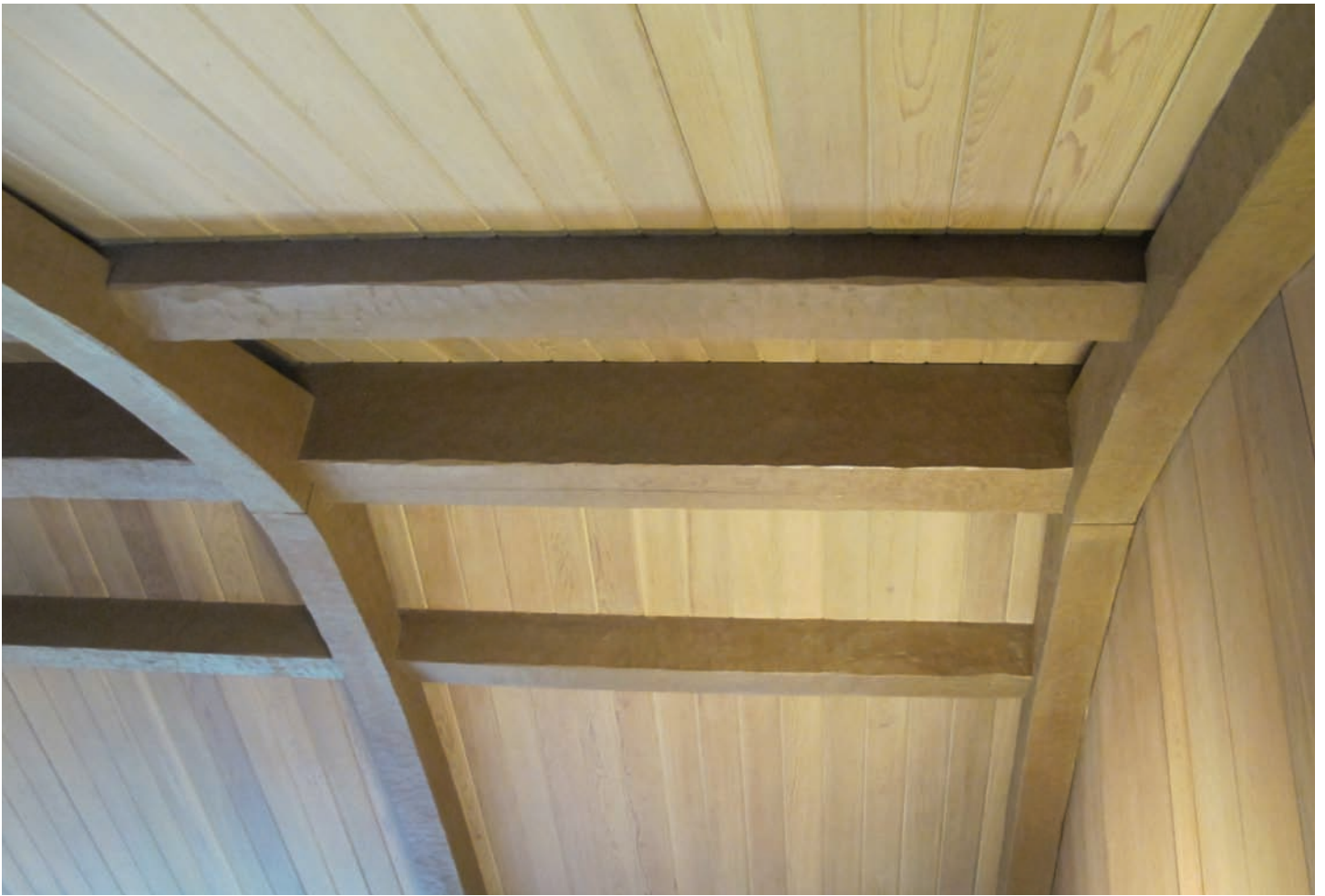
Living room ceiling detail
