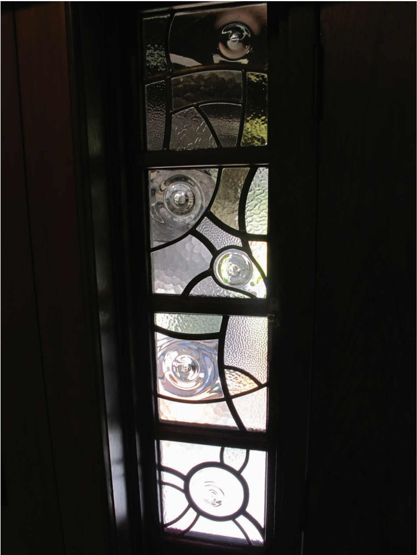
Side light detail, front entrance
