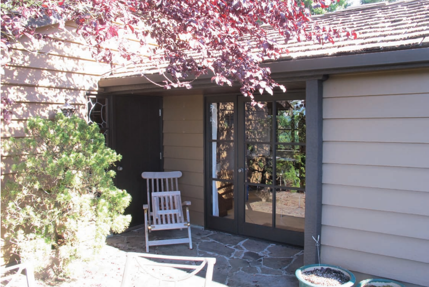
Rear patio and access to kitchen
