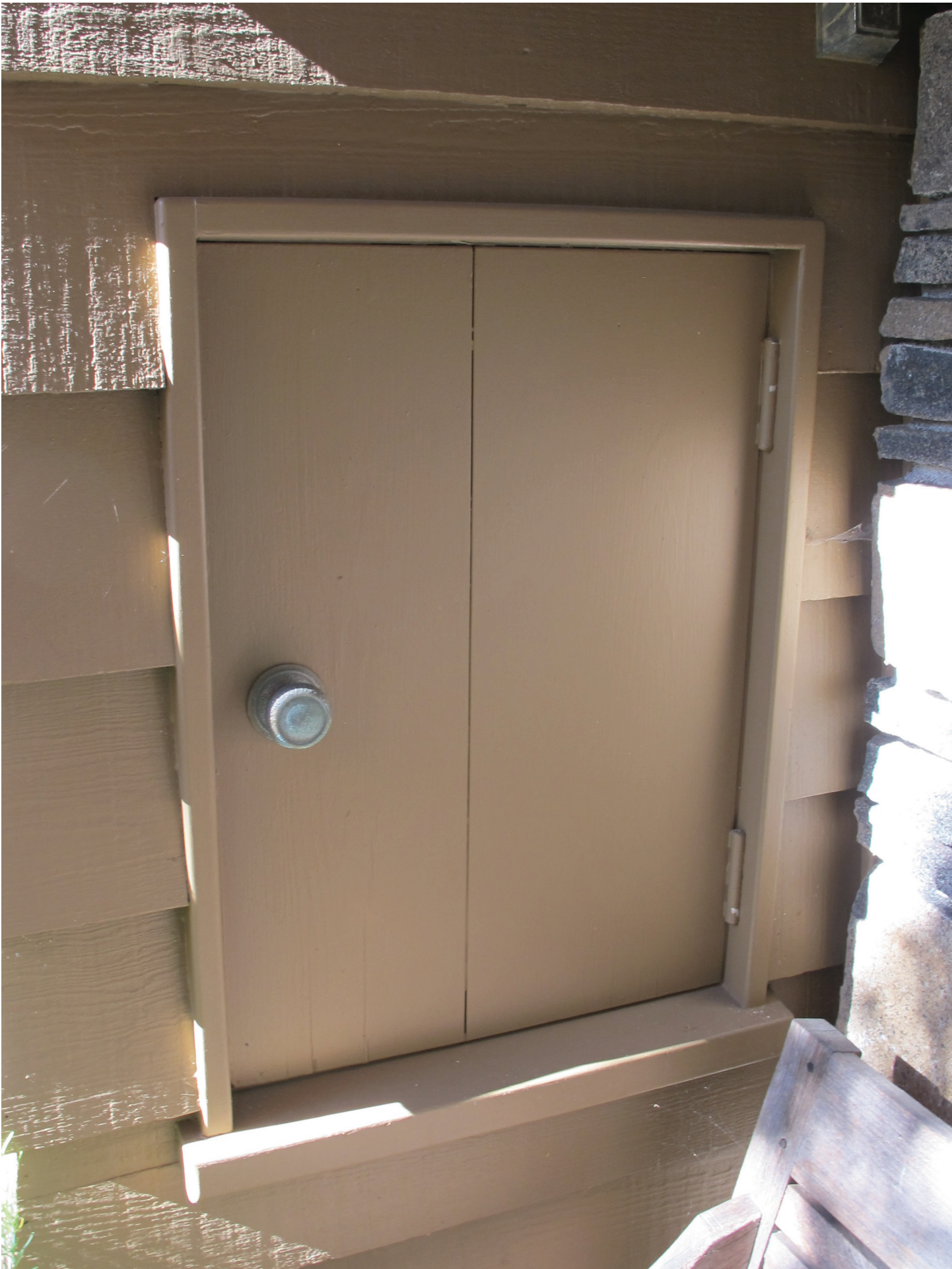
Access door on exterior for service deliveries
