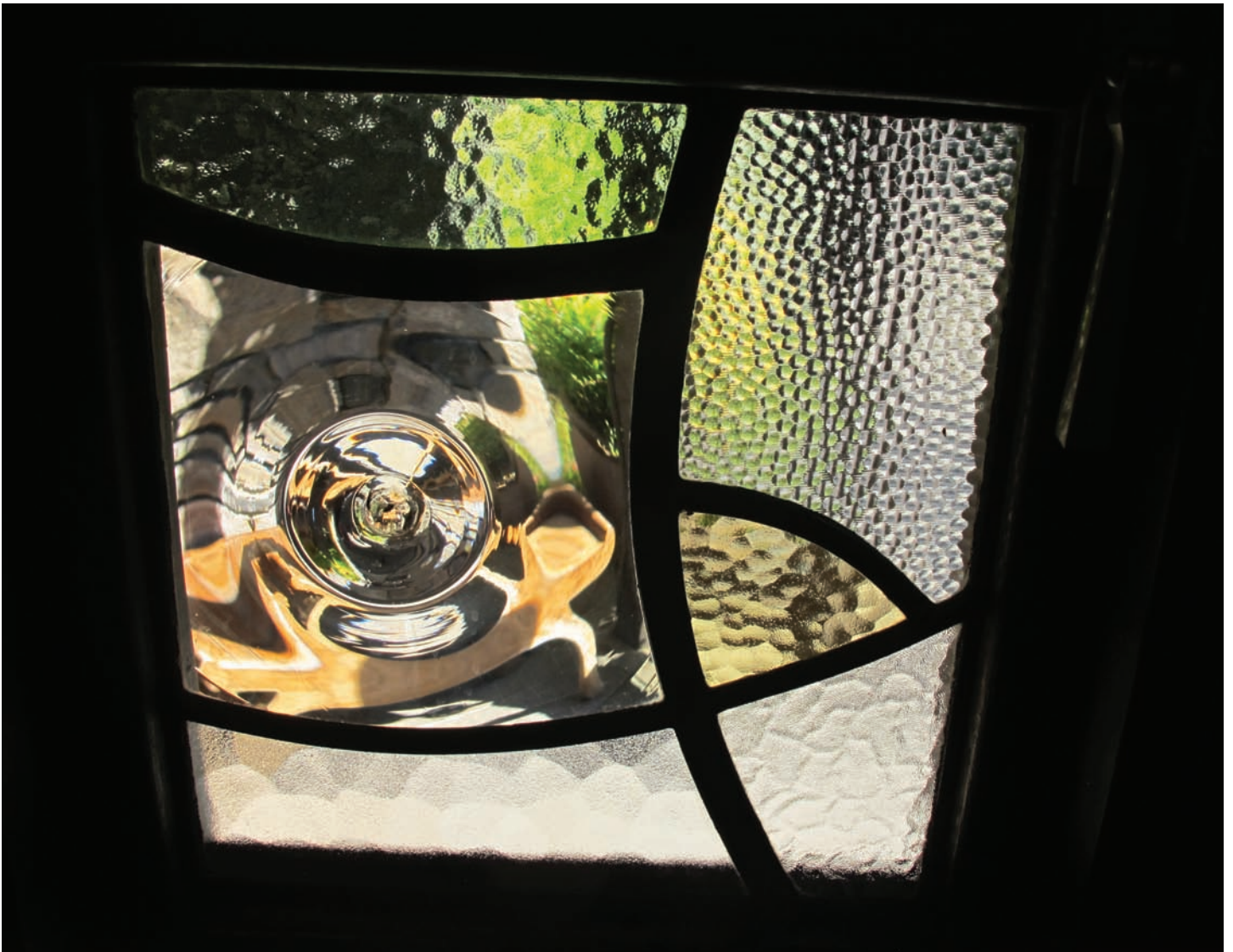
Window detail, front entrance side light
