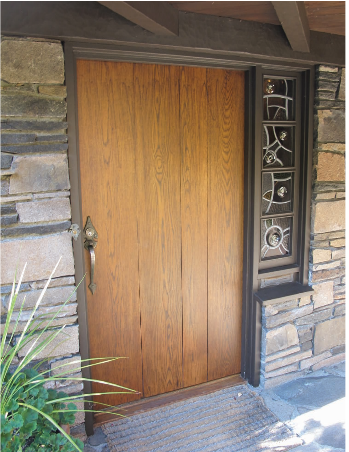
Front entrance detail
