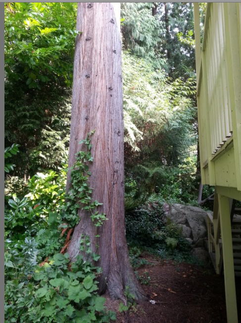
Photo 4. Several trees are growing within the existing building's envelope. Note these trees should be removed before house demo.
