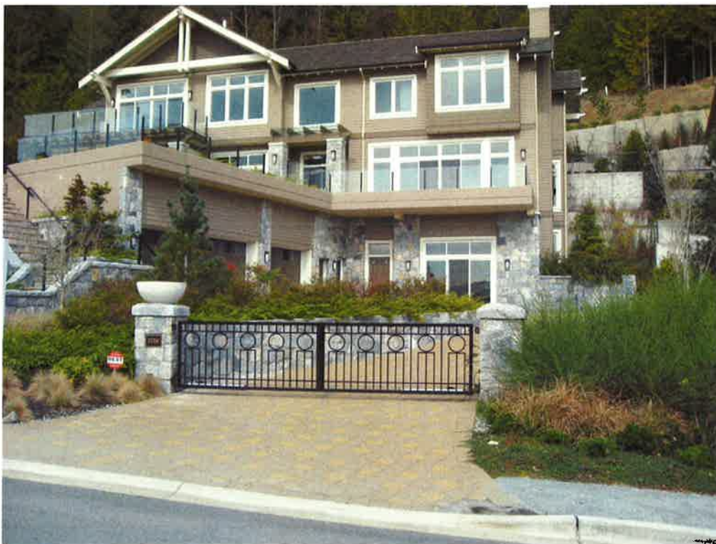
Uphill House – Variances Allowed – flat driveway, “eyes on street”, retaining walls hidden by house
