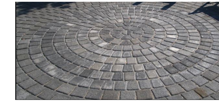
entry courtyard - concrete unit paver
