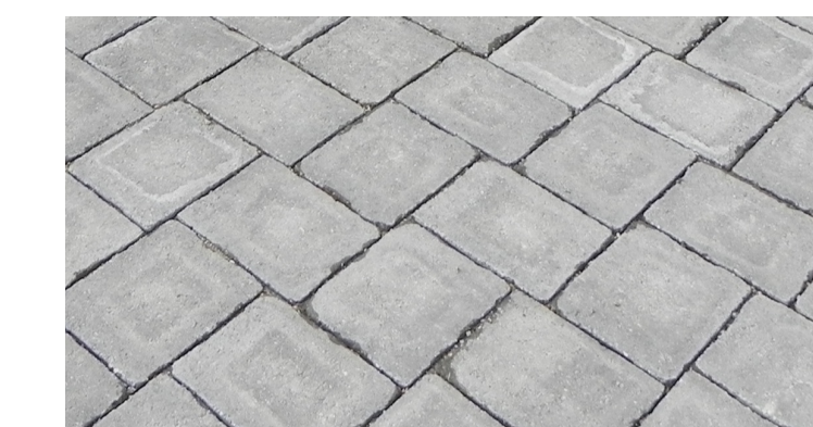
driveway - permeable paver
