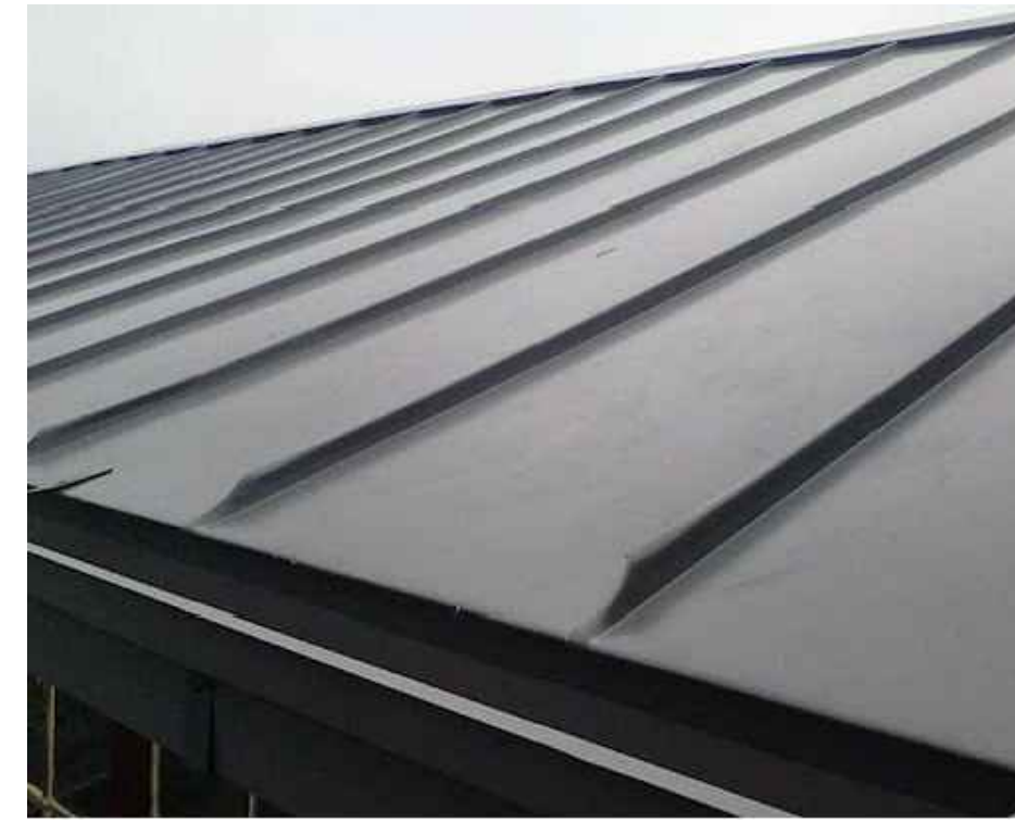
UP-STAND SEAM METAL ROOFING GRAY
