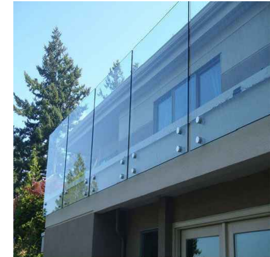
CLEAR TEMPERED GLASS RAILING (SIDE MOUNT)
