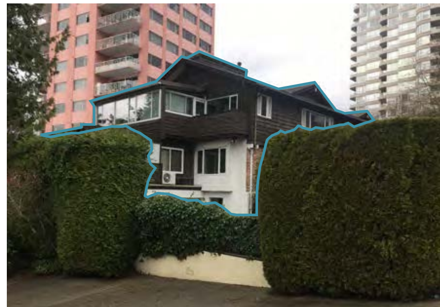
E) View from south east corner of site
