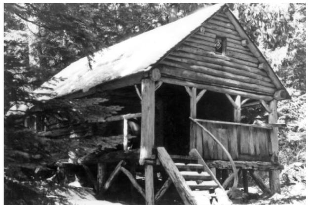
*Fig 4 Pastime (240)* Log structure, cedar shake peak roof
