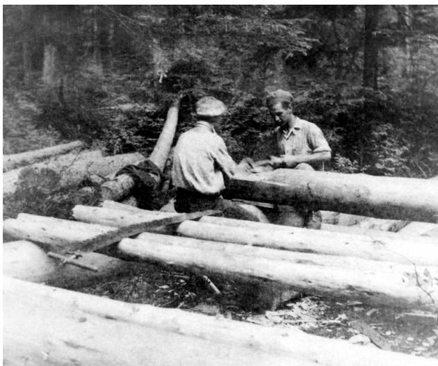
*Fig 7* Making a joint. These are floor strings that the saw is on
