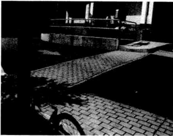
BAD No curb cut at crossing area.
