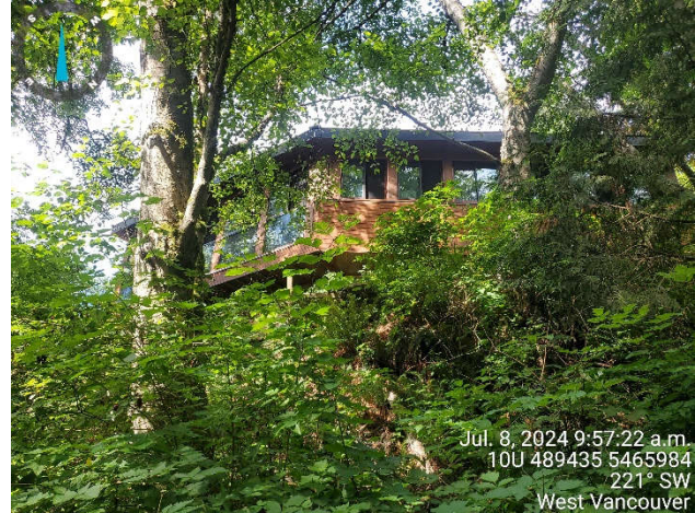
Photo 6: View of the unpermitted building from the stream boundary of Brothers Creek.
