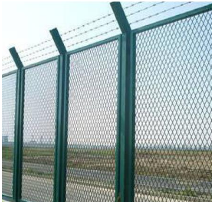
Figure 2 – Option B – expanded metal fence with barbed wire on top
