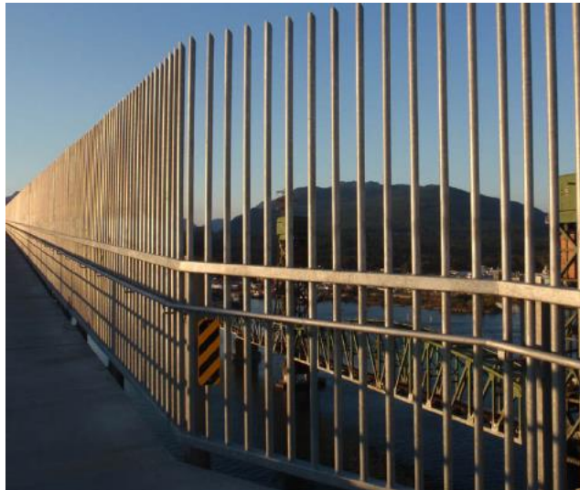
Figure 3 – Option C - specialized barrier on Second Narrows Bridge
