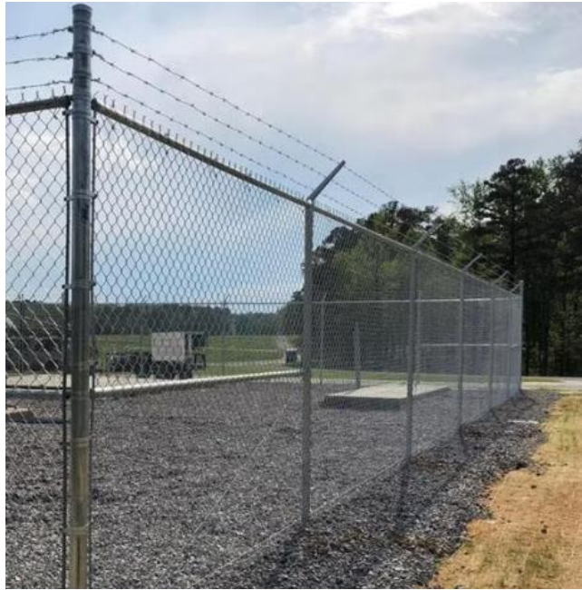
Figure 1 – Option A - chain-link fence with barbed wire on top
