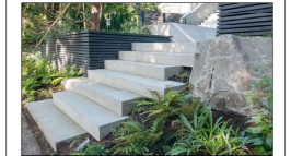
CONCRETE PAVERS WITH BOULDERS AND GROUNDCOVER
