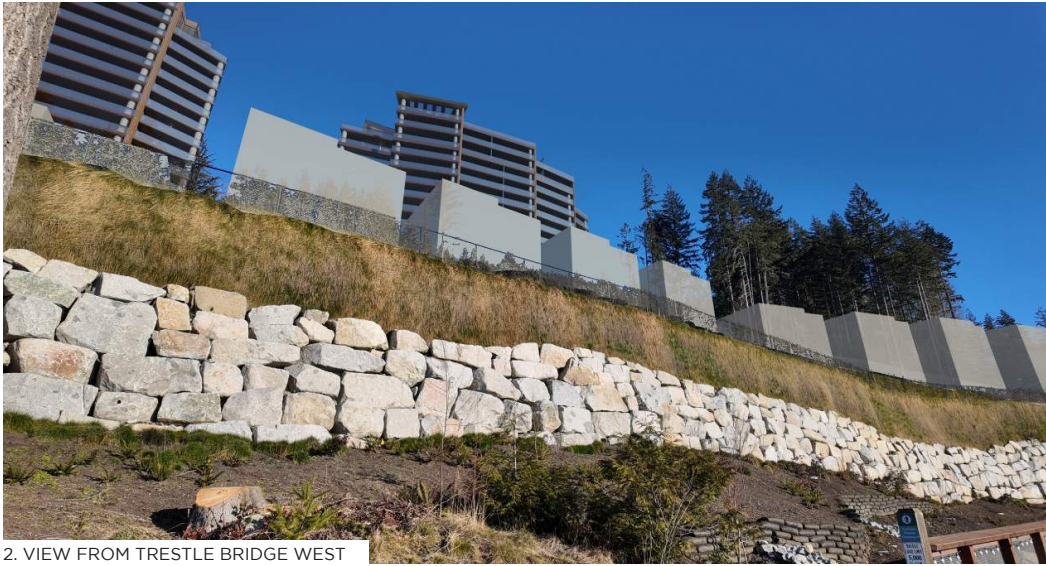
2. VIEW FROM TRESTLE BRIDGE WEST
