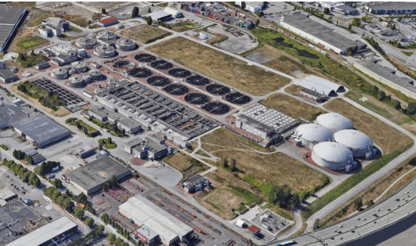
Annacis Island WWTP: ~50 hectares
