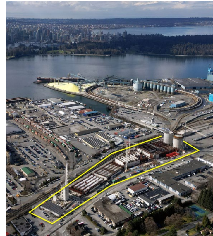
North Shore WWTP: 3.5 hectares
