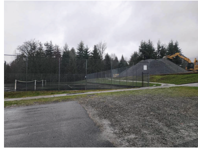
EXISTING TENNIS COURT LOOKING NORTH WEST
