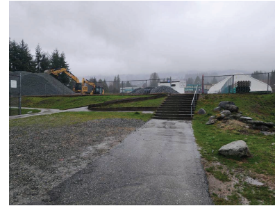
EXISTING STAIRS LOOKING NORTH
