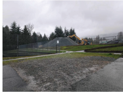
EXISTING TENNIS COURT LOOKING NORTH WEST
