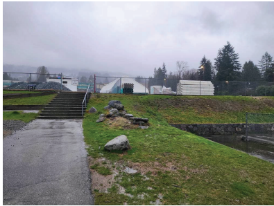
EXISTING STAIRS LOOKING NORTH
