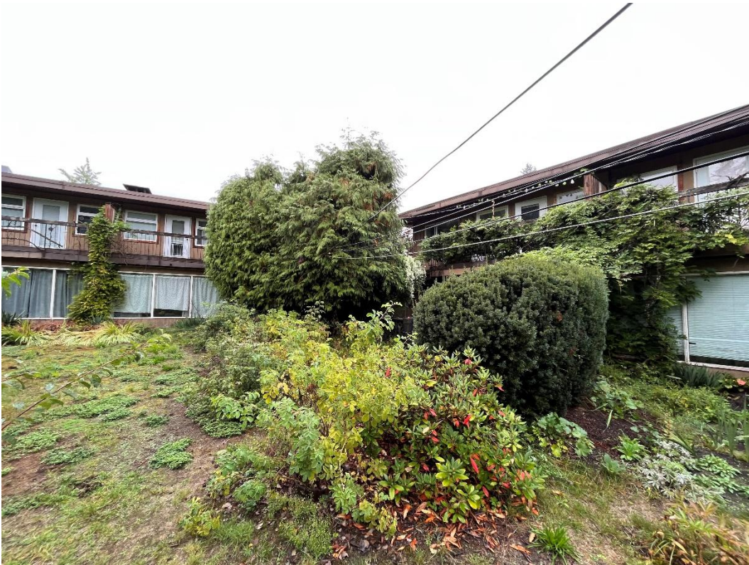
Photo 2. Protected tree #1895 recommended for removal to maintain fuel free buffer (middle).
