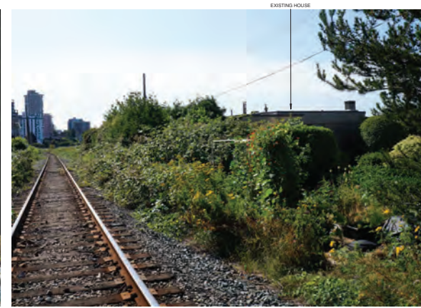
VIEW OF EXISTING HOUSE FROM RAILROAD
