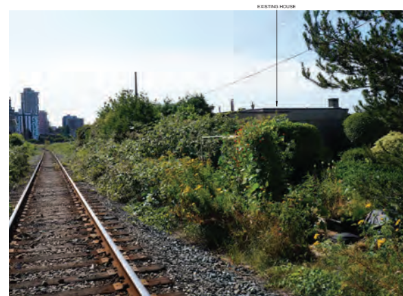
VIEW OF EXISTING HOUSE FROM RAILROAD
