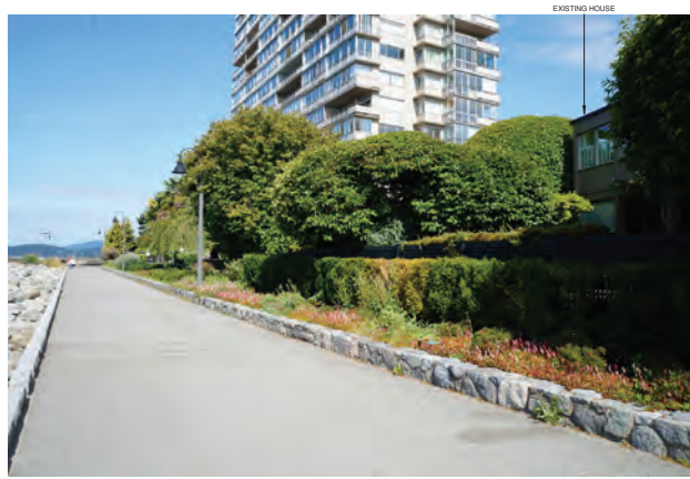
VIEW OF EXISTING HOUSE + SEASTRAND BUILDING FROM SEAWALK
