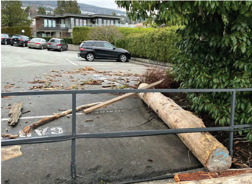
Figure 3-7. Flood evidence on the parking lot west of the project site - facing northeast.
