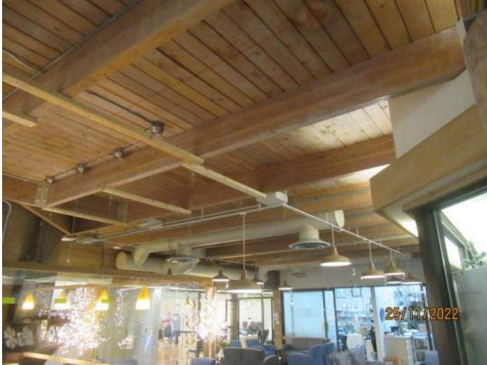
Typical Interior Framing – 1980 Construction
