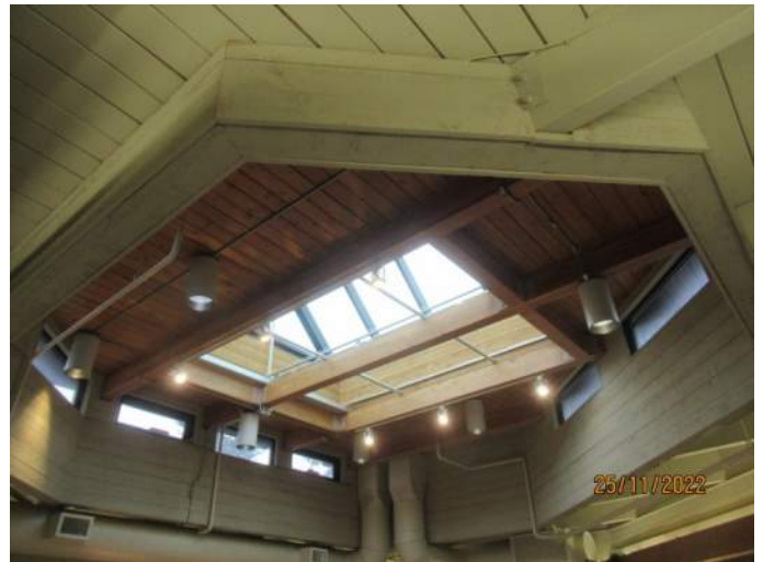
Typical Interior Framing – 2001 Construction
