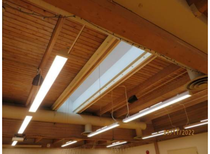
Typical Interior Framing – 1980 Construction
