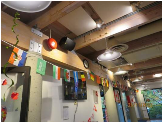
Typical Interior Framing – 2001 Construction
