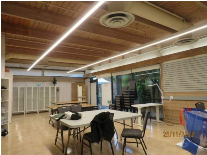
Typical Interior Framing – 1994 Construction
