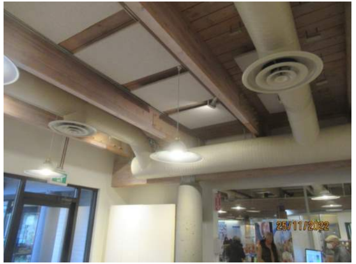
Typical Interior Framing – 1994 Construction
