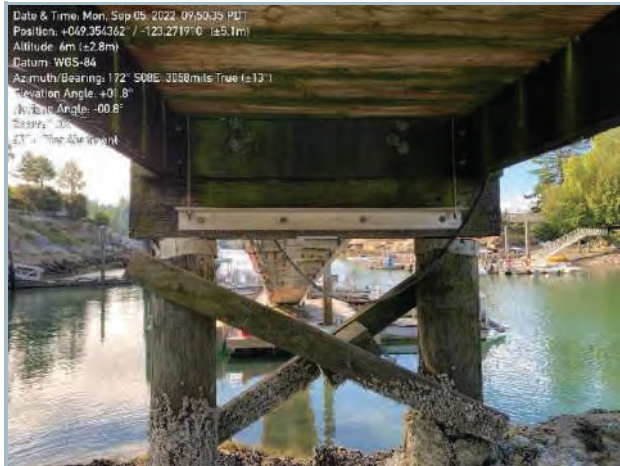
020. Gangway Access Platform to Timber Pier Connection
