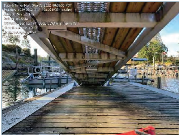
011. Aluminum Gangway Soffit Viewing South
