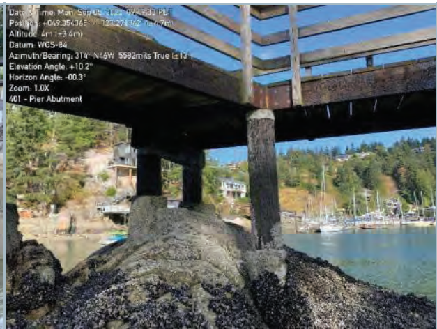
010. West Pier Abutment on Bedrock
