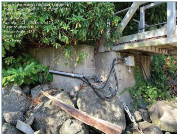
007. Southwest Abutment Wingwall
