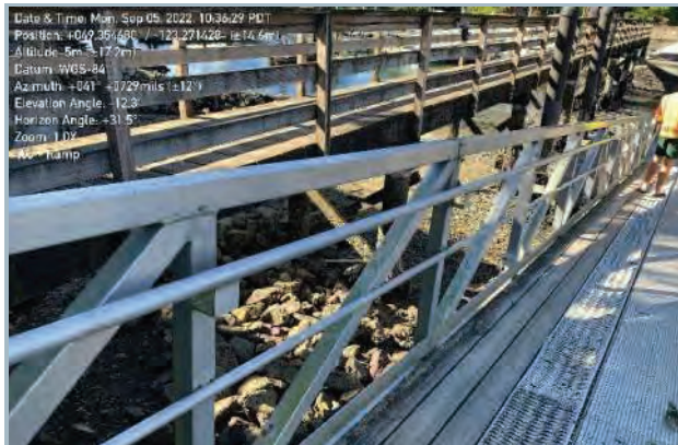
007. Gangway Railing & Truss Orientation
