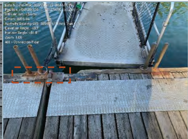
035. Overlapping Plates at Dock Connection
