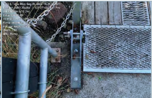
008. Gangway Connection to East Abutment
