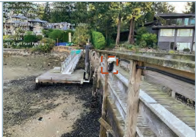
029. Diminishing Black Paint on Light Fixtures, Typ.
