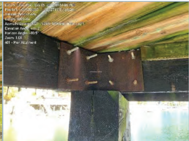
019. Interior Bolted Angle Connection
