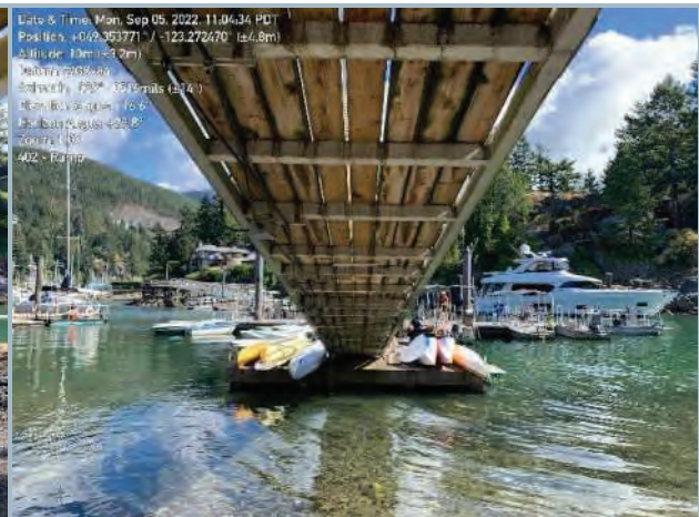
012. East Segment Gangway Soffit
