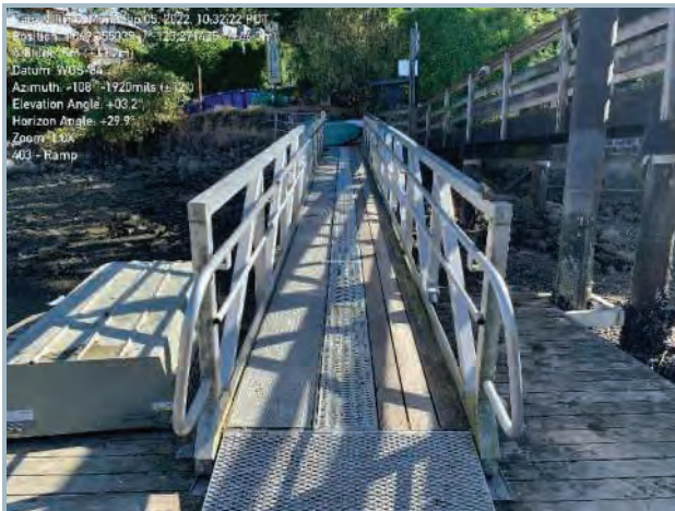
003. East Approach Gangway Viewing East
