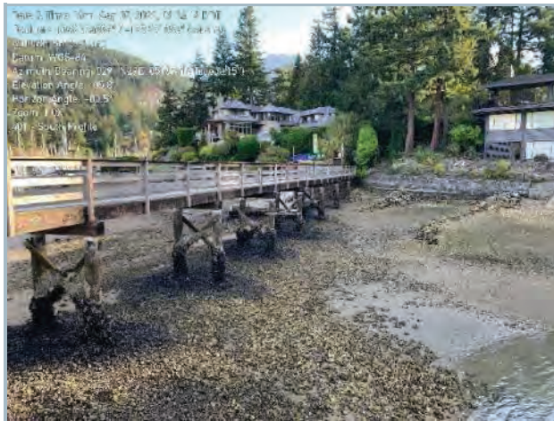
009. Braced Timber Piers, Typ.
