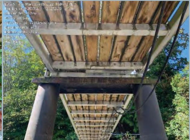
006. Steel Pile West Pier
