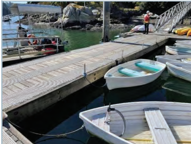
009. Deck of East Intermediate Landing Dock
