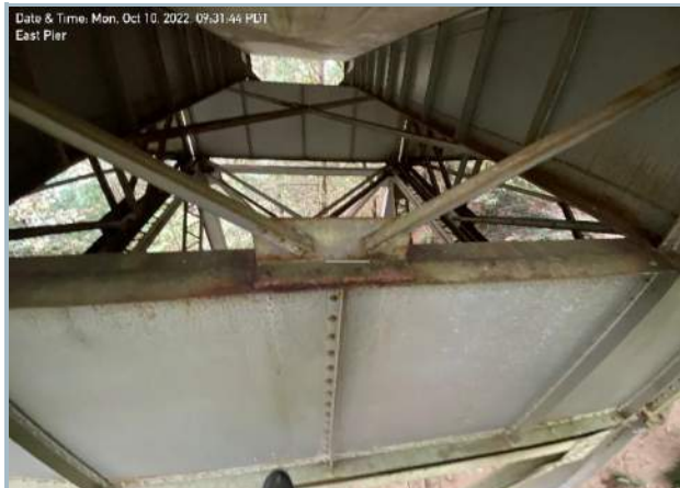
032. Alternating Longitudinal Bracing Along North Profile, Typ.
