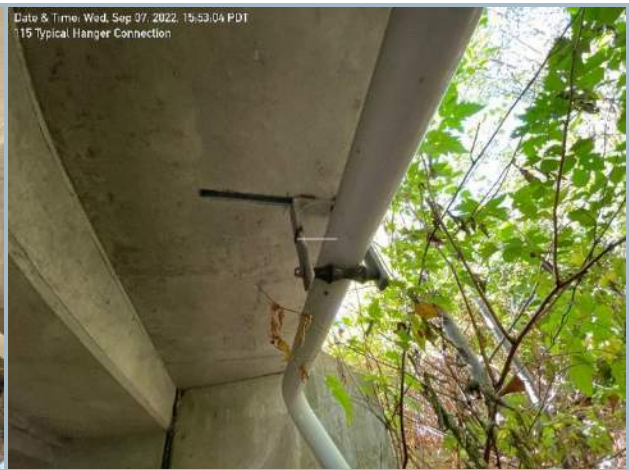
014. Utility Line Along North Profile
