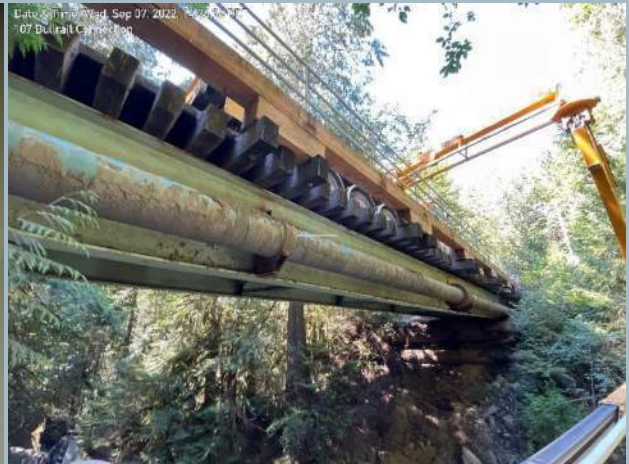
014. Watermain Utility Along East Profile
