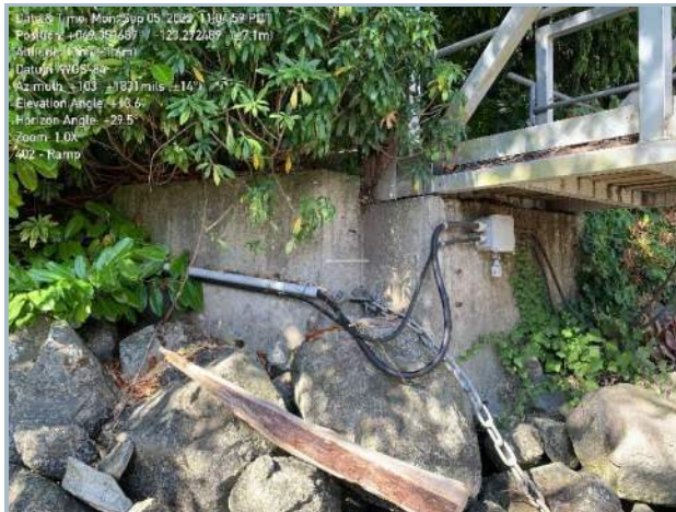
007. Southwest Abutment Wingwall
