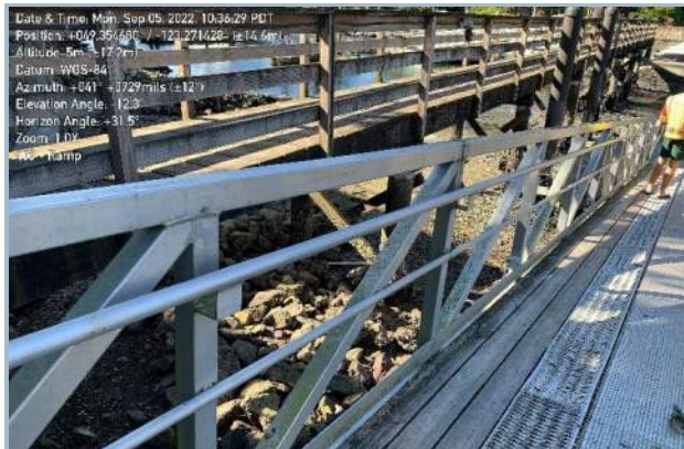
007. Gangway Railing & Truss Orientation
