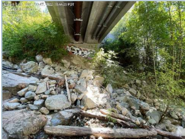
013. East Embankment (Note Debris Accumulation in Creek Bed)
