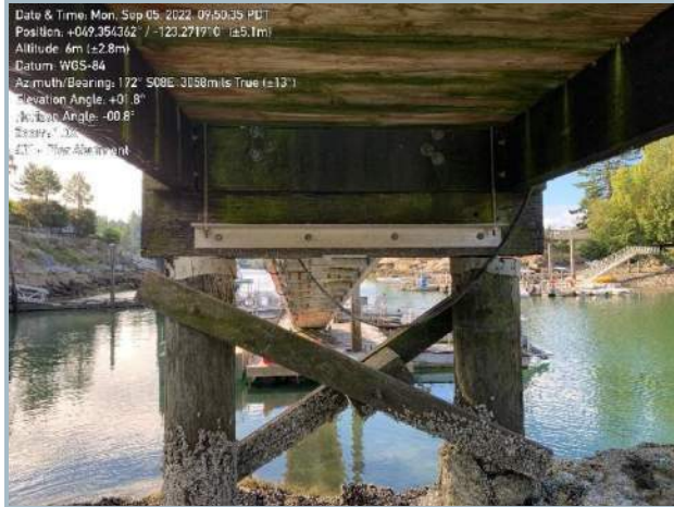
020. Gangway Access Platform to Timber Pier Connection
