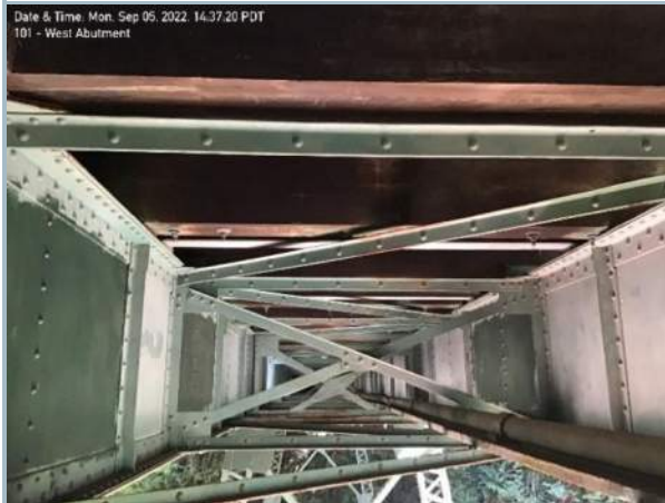
021. Cross-Bracing Elements of Riveted Steel Plate Girders, Typ.
