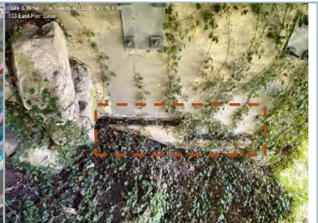
022. Reinforced East Pier Base
