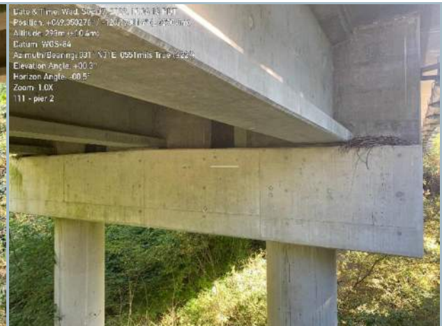
022. East Pier Pile Cap
