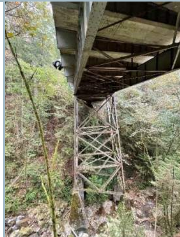
010. East Pier Abutment
