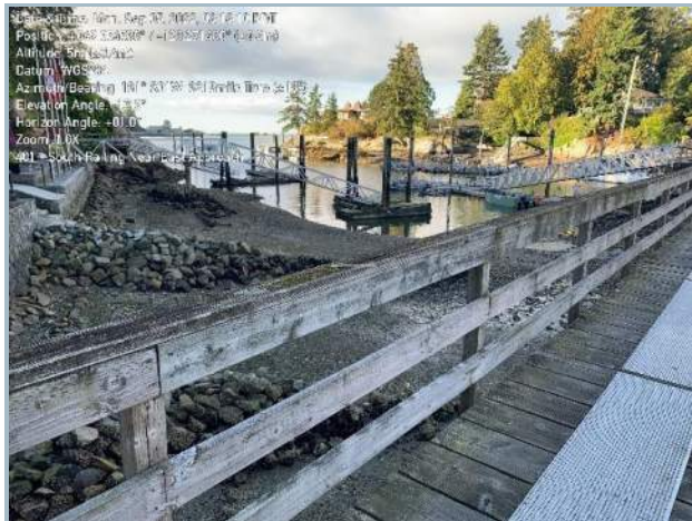
013. Timber Railing, Typ.
