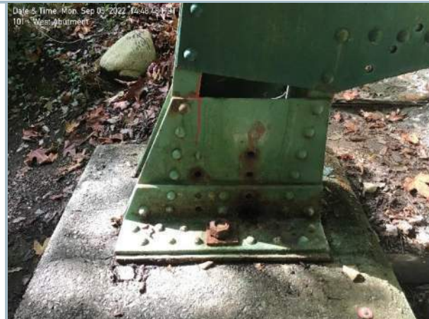
022. Anchored Pier Footing Connection, Typ.
