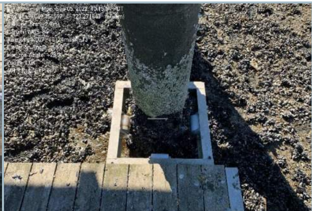
010. Dock Restraint Timber Pier Connection
