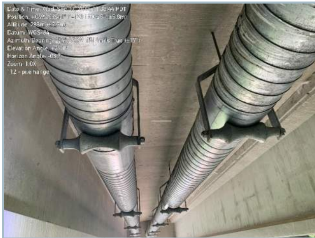
015. Utility Pipes Along South Interior Section
