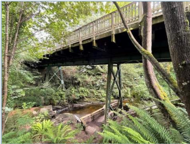
003. North Elevation Viewing East
