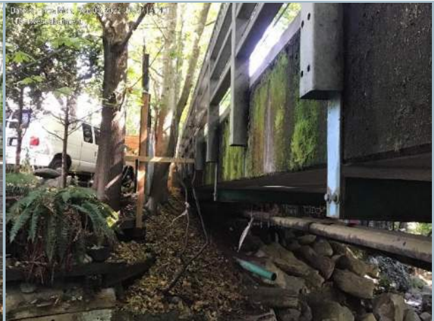
012. Railing Connection, Typ.
