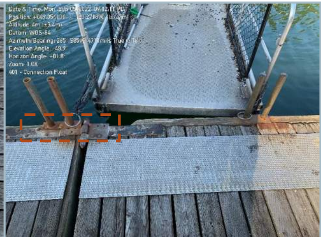
035. Overlapping Plates at Dock Connection
