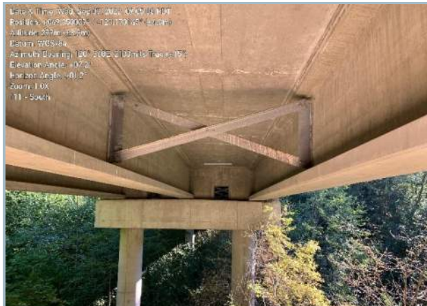
103. Lateral Bracing at Midspan, Typ.
