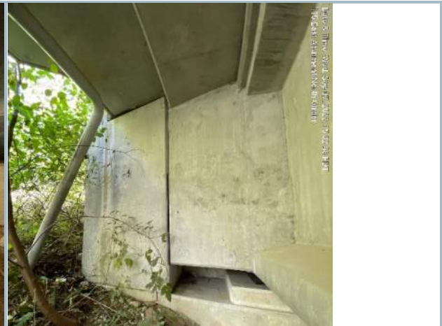
018. North Girder Shear Key at East Abutment
