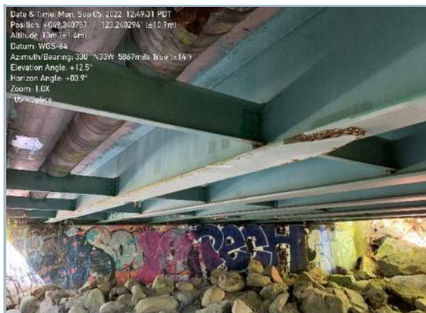
016. Stringer Welded Strengthening Plate at Midspan Sections, Typ.
