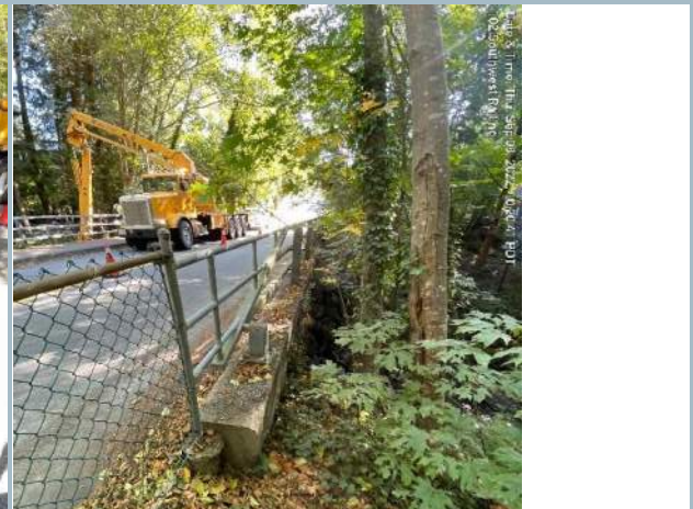
016. Northwest Railing Transition
