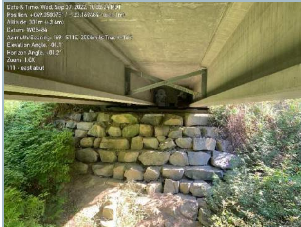
007. East Abutment (Note Boulder Embankment with Geogrid)
