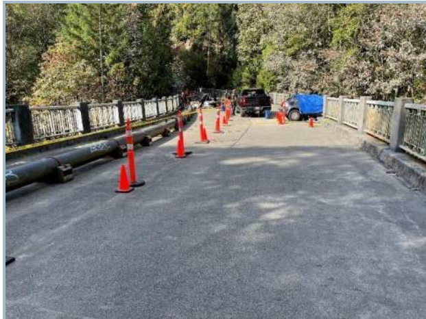
011. Bridge Deck Viewing West
