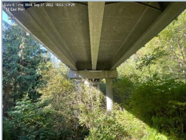
009. East Pier Abutment
