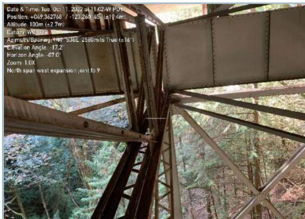
034. Vertical Bracing over Pier Section, Typ.
