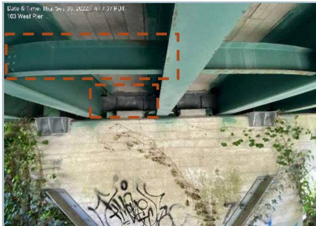
017. Intermediate and Pier Lateral Restraint (As part of Shear Key Retrofit)
