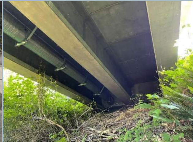
010. Bridge Soffit (Note Precast Deck Panels)
