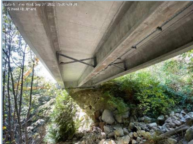
019. Midspan Lateral Bracing Members, Typ.
