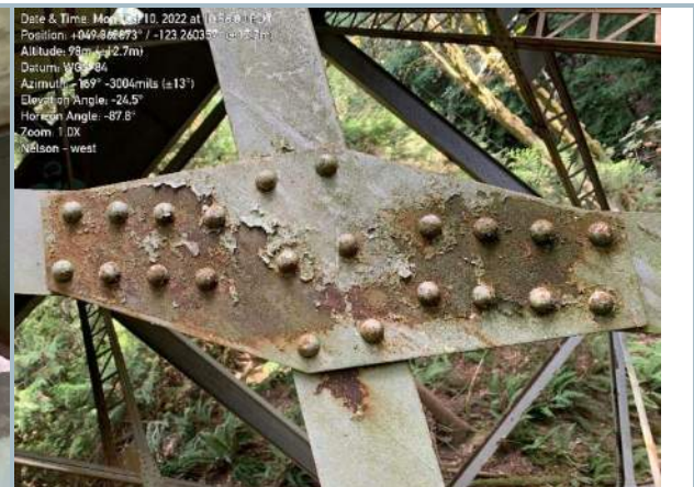
205. Pier Cross-bracing Connection, Typ.
