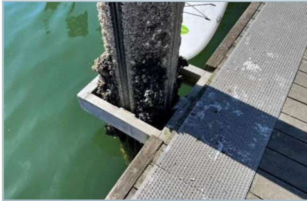
013. Exterior Dock-Timber Pile Restraint Connection, Typ.
