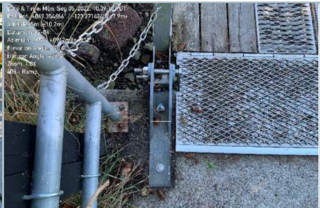
008. Gangway Connection to East Abutment
