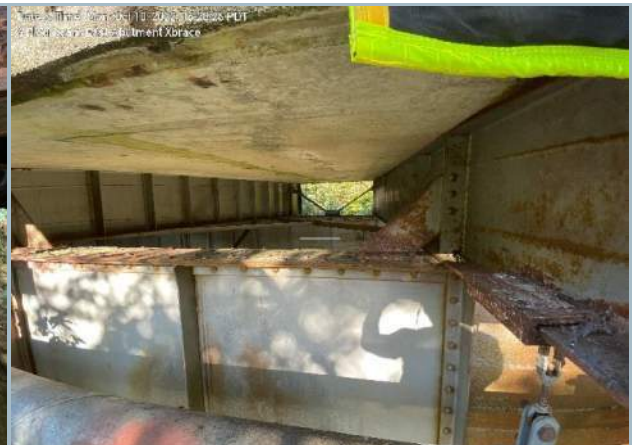
031. Alternating Knee Bracing along South
