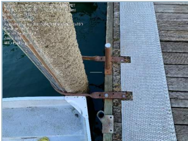
034. Dissimilar Timber Pile Restraint
