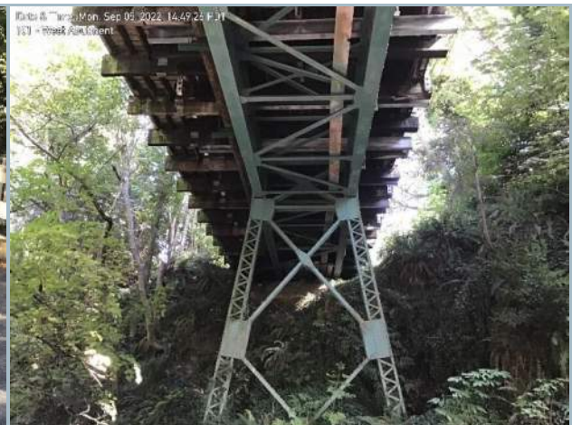
012. Bridge Soffit Viewing East
