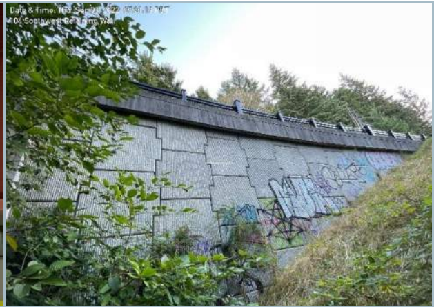
012. MSE Retaining Wall Along Southeast Section, Typ.
