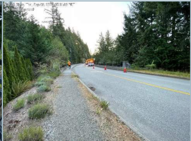
006. West Approach (Note Skewed Orientation)
