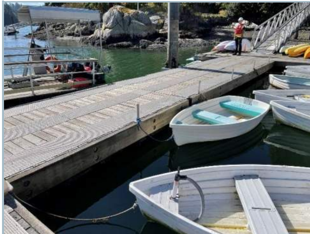
009. Deck of East Intermediate Landing Dock
