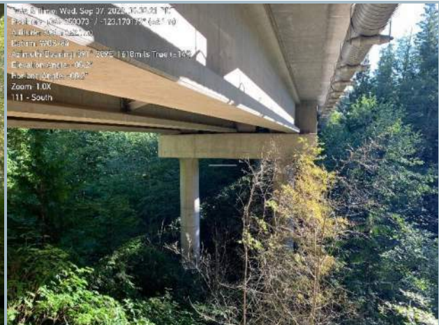
010. West Pier Abutment
