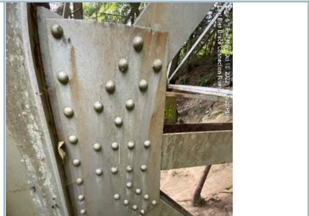
019. Pier Lateral Bracing Gusset Plate Connection, Typ.
