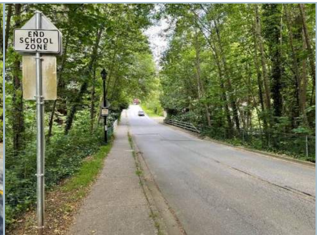
006. West Approach (Note Sidewalk along North Profile)
