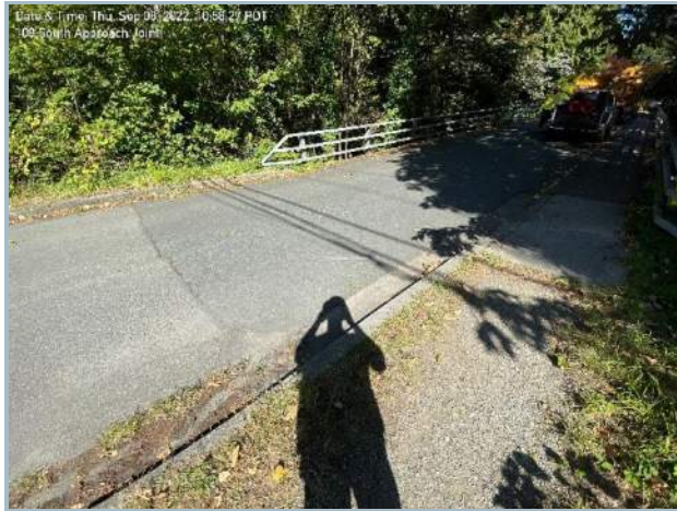
011. South Approach Slab Joint
