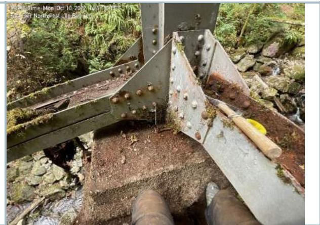
203. Pier Corner Connection, Typ.
