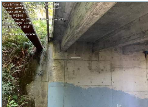
017. Precast Concrete Stringers with Integral Abutment and Concrete Deck Diaphragm
