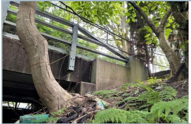
015. Prestressed Box Girders Bearing on Semi-Integral Abutment
