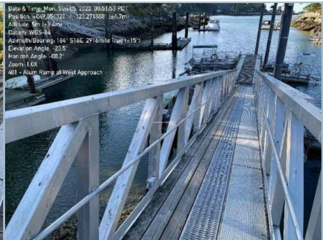
014. Aluminum Gangway Truss Rail, Typ.
