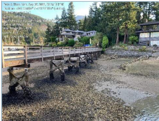
009. Braced Timber Piers, Typ.
