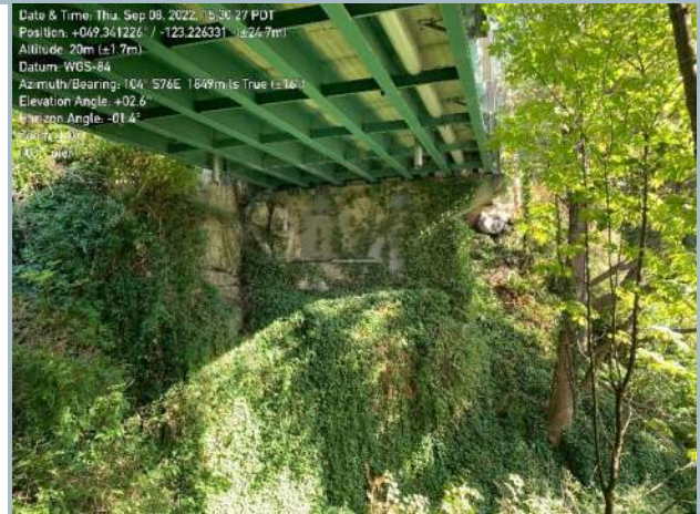
010. East Pier Abutment
