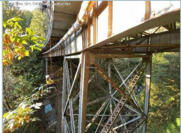
004. South Elevation (Note Existing Utility Pipe)
