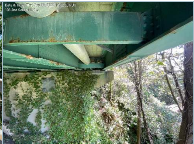
014. Utility Along South Profile
