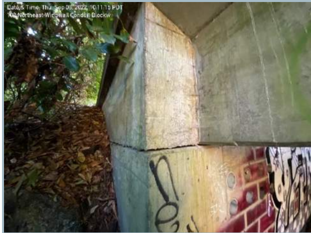
018. Northeast Integral Wingwall, Typ. (Note: Conduit Voids)
