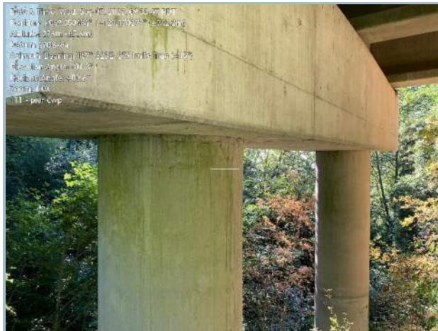
021. West Pier Pile Cap
