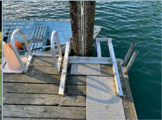
021. Timber Pile Dock Restraint Connection, Typ.
