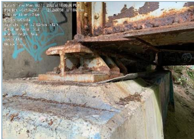
030. Anchored Bearing Plate Connection
