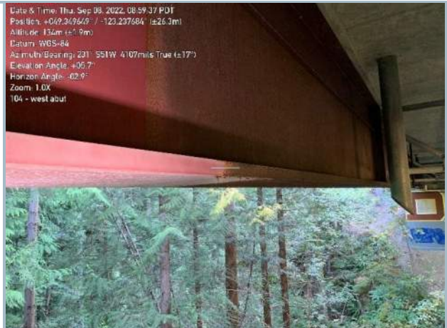
016. Change of Girder Coating Near Abutments, Typ.
