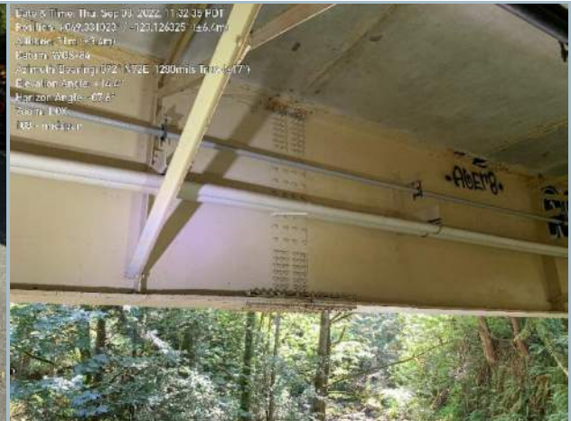
018. Girder Splice Connection, Typ.
