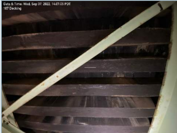
013. Deck Soffit with Transverse Beams
