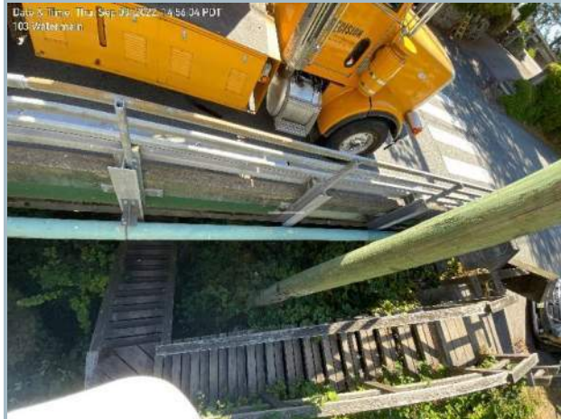
015. Sanitary Utility along North Profile (Note: Park Entrance at Northwest Section)
