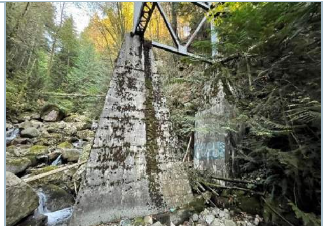
015. Northwest Pier Pedestals at East End
