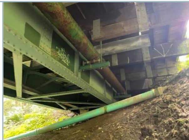
018. Utility Transversely Crossing West Abutment (Note Timber Deck)
