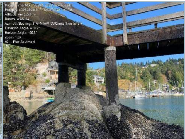
010. West Pier Abutment on Bedrock
