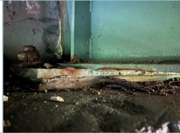
020. Anchored Bearing Plate Connection, Typ.
