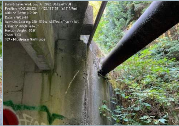
014. Utility Lines at North Profile
