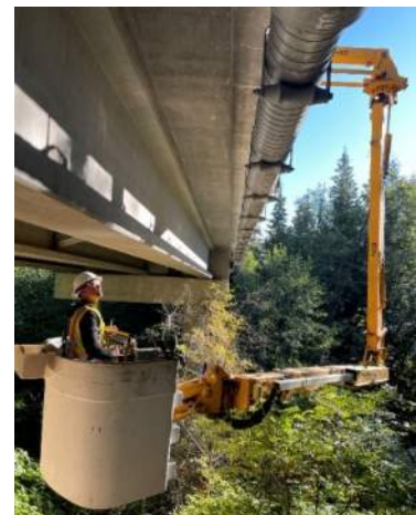
Figure 2. UBIV Inspection Access
