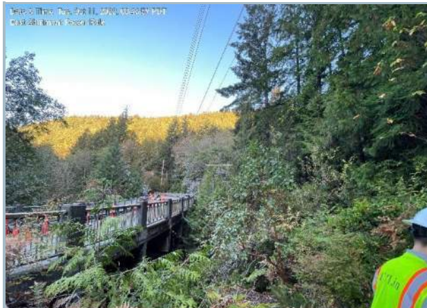
028. Utility Power Line Viewing from East Abutment
