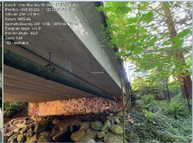
012. Bridge Soffit Viewed from South Profile
