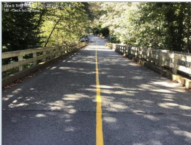
011. Bridge Deck Viewing West
