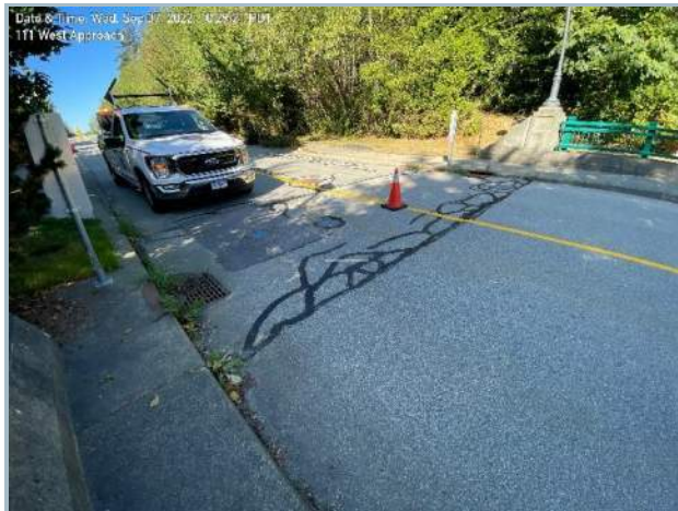
019. West Approach Slab Joint
