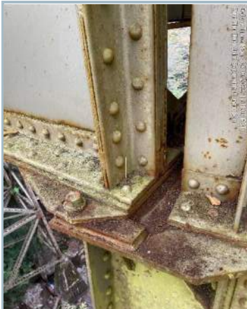
018. Girder Connection to Accommodate Bridge Skew, Typ.
