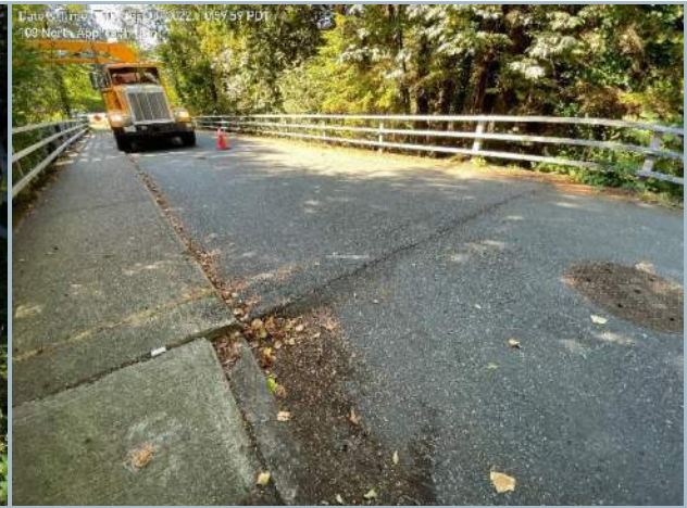
012. North Approach Slab Joint
