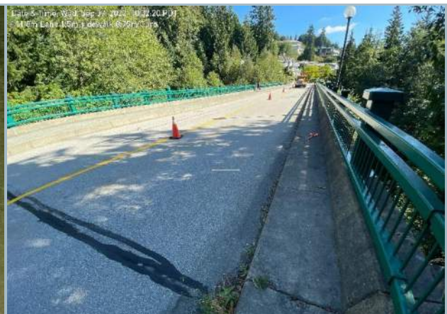
018. Sidewalk along North Profile and Boulevard along South Profile
