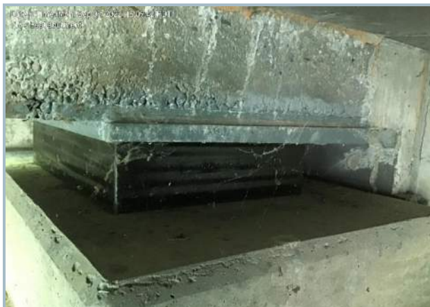
015. Shear Key at Abutment
