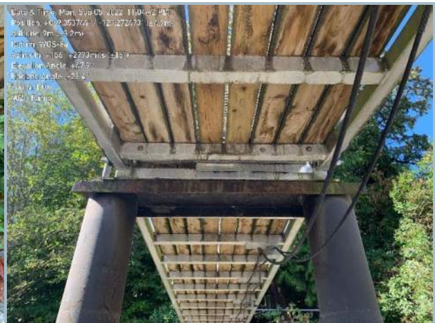
006. Steel Pile West Pier
