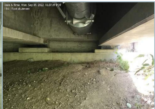
016. Transverse Lateral Restraint along Backwall
