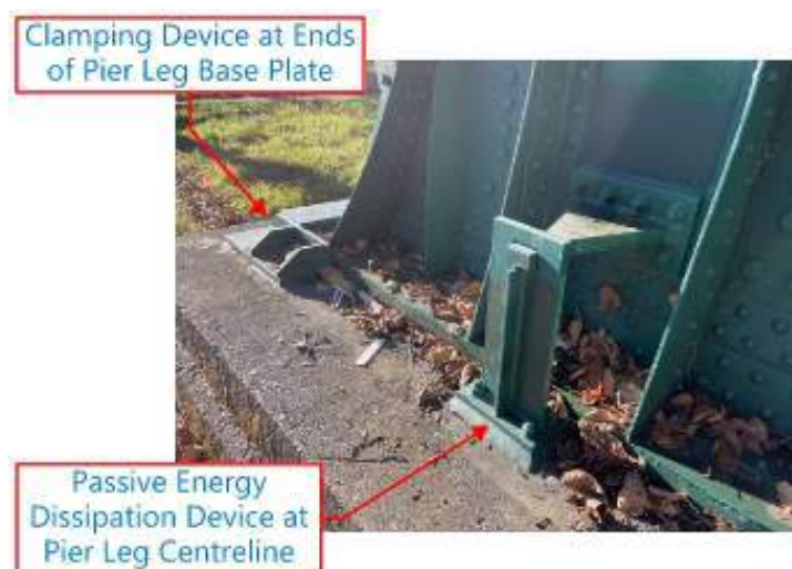
Figure 5. Typical Rocking Connection Components on the Lions Gate Bridge Approach Spans
