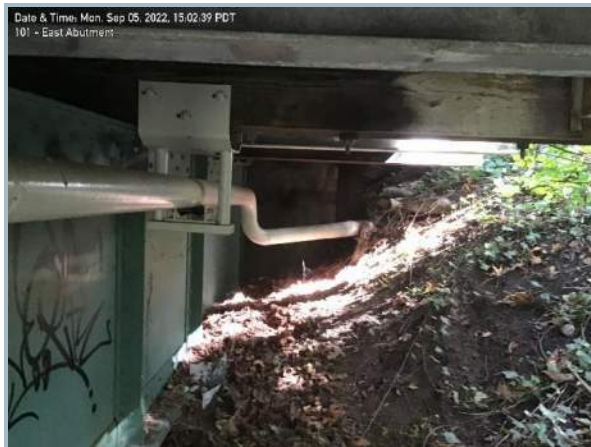
017. Gas Utility at Southeast Section of East Abutment
