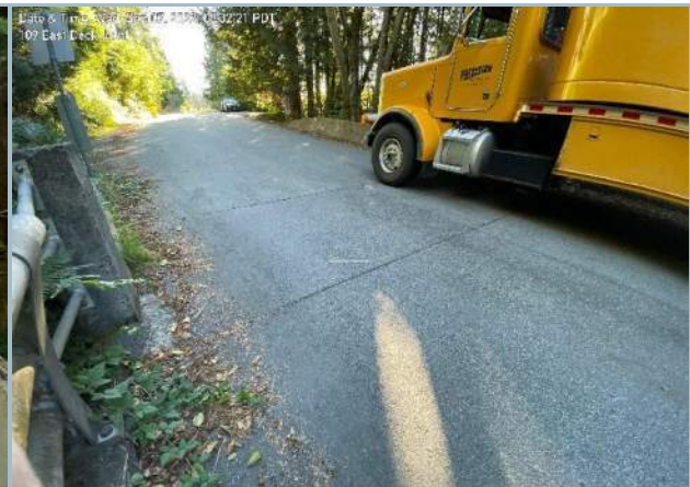
016. East Approach Slab Joint
