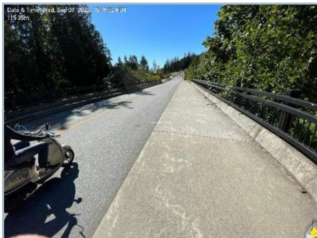
015. Sidewalk Along North Profile
