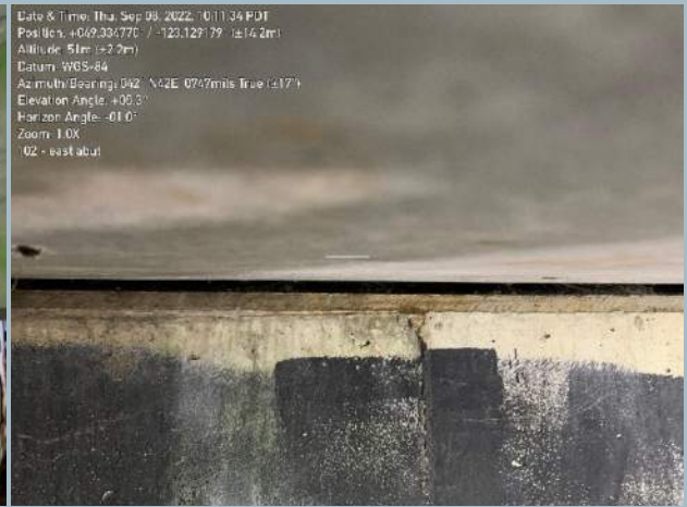
019. Elastomer Bearing at Abutment, Typ.
