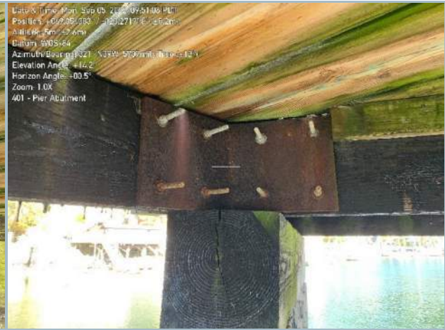
019. Interior Bolted Angle Connection
