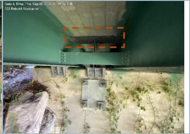
020. Longitudinal Diagonal Restraint System at East Pier, Typ.
