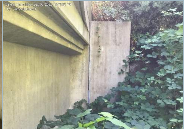
013. Wingwall at West Abutment
