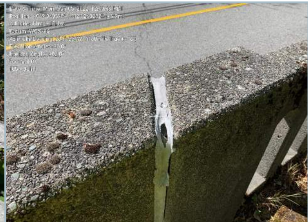
015. North Parapet Joint
