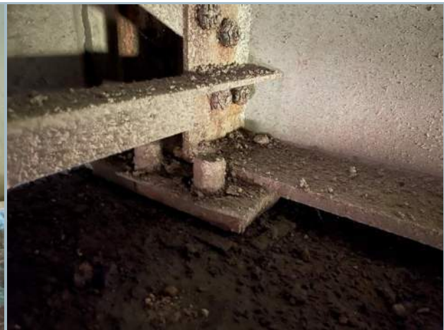
017. Anchored Steel Bearing Plate, Typ.
