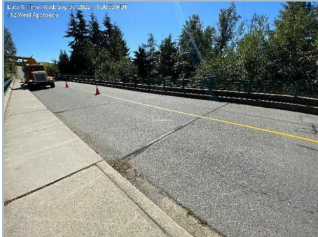
009. Bridge Deck (Note West Approach Slab Joint)
