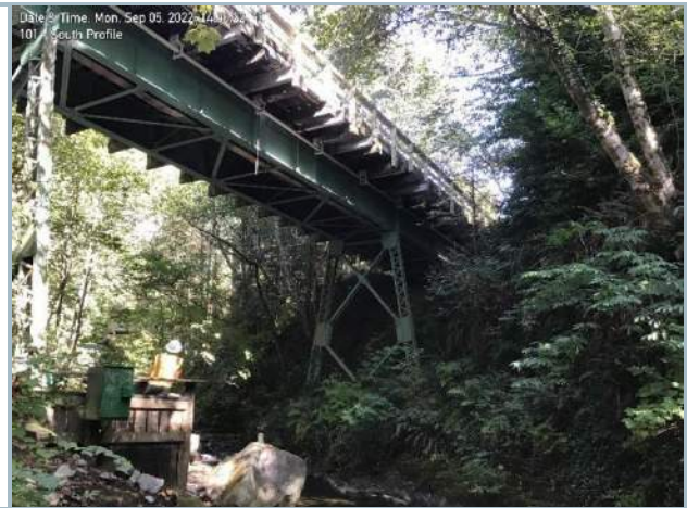
010. East Pier Abutment
