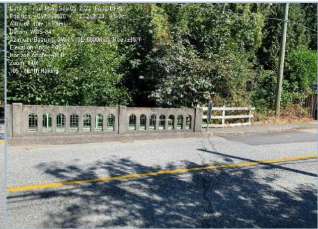
013. North Parapet and Pedestrian Walkway
