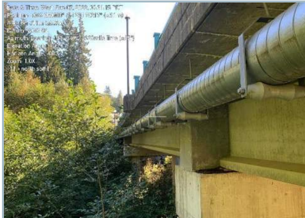
015. Utility Pipe Along South Profile
