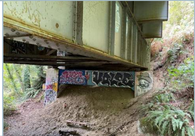
017. Jump Span Cap Beam at West Abutment
