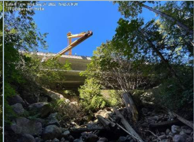
004. South Elevation (Note: Downstream Debris in Creek Bed)
