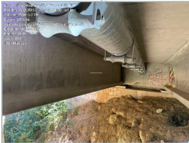
013. Interior Waterman Utility
