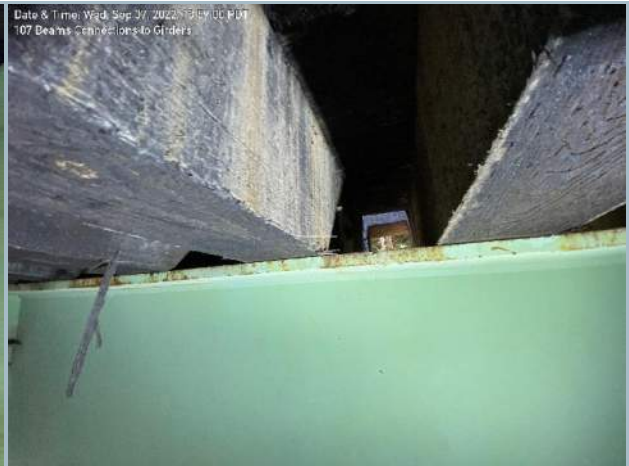
012. Transverse Beams Bearing on Steel Girders
