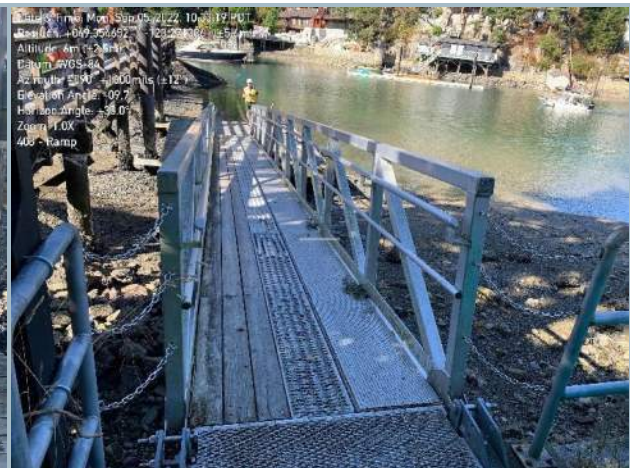
004. East Approach Gangway Viewing West
