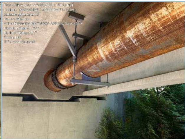
016. Utility Pipe Along North Interior Section
