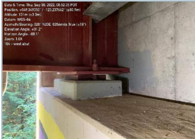
019. Anchored Elastomeric Bearing at Abutment, Typ.
