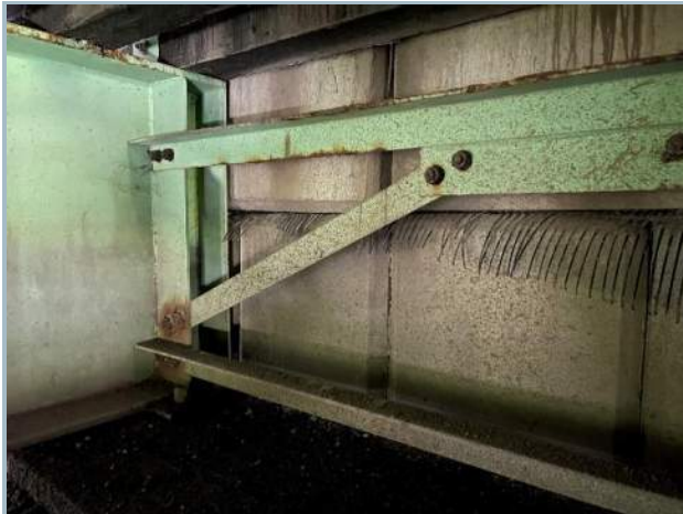
007. South Abutment (Note: Lock block Back Wall, Typ.)
