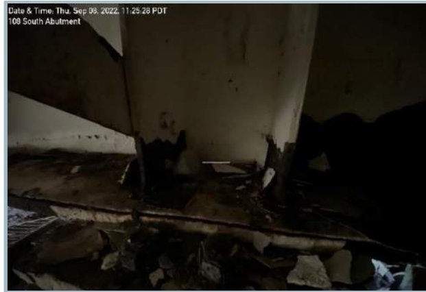
015. Coating Failure at Bearing Plate of South Abutment
