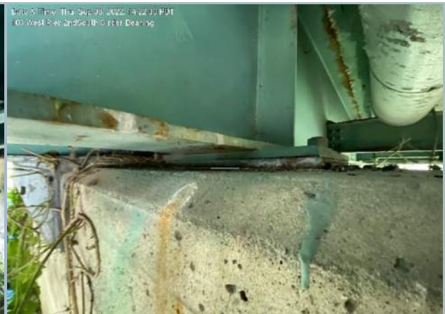
018. Anchored Steel Bearing Plate, Typ.
