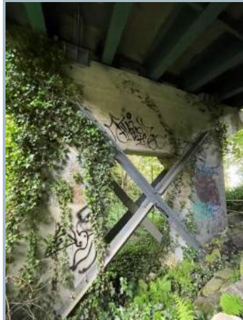
009. West Pier Abutment
