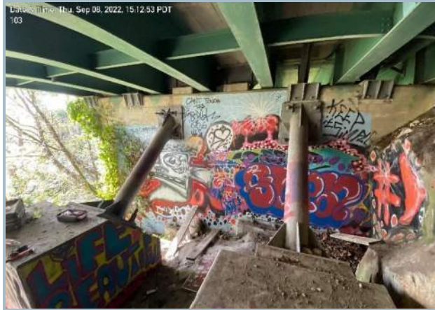
019. Longitudinal Anchor Restraint System at East Pier
