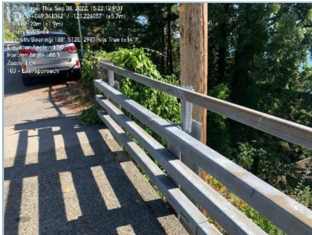
013. South Railing Detail, Typ.
