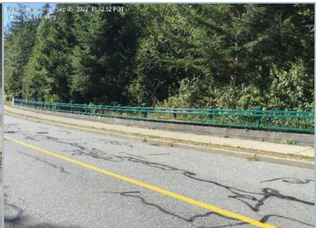
014. North Railing, Typ.
