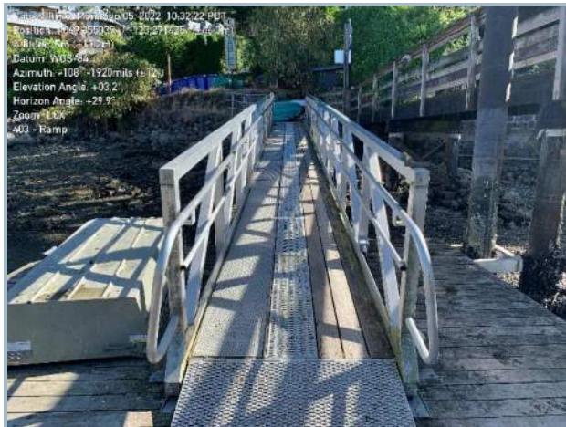
003. East Approach Gangway Viewing East
