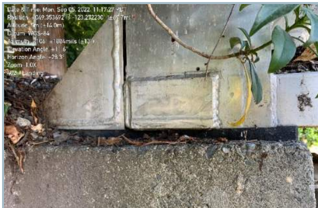
015. Shear Key at Abutment
