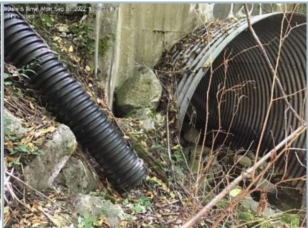
016. Stormwater Drainpipe East of Culvert Inlet
