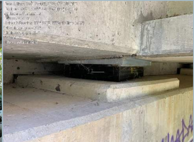
020. Elastomeric Bearing Pad in Moderate Condition, Typ.
