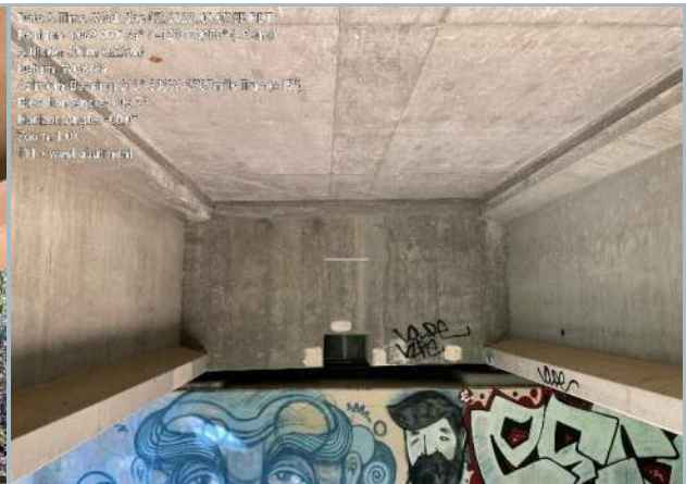
104. Shear Key at Pier Abutment, Typ.
