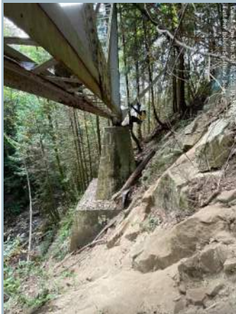
016. Southeast Pier Pedestal at West End
