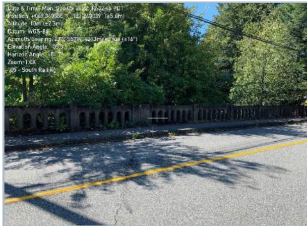
012. South Parapet and Sidewalk
