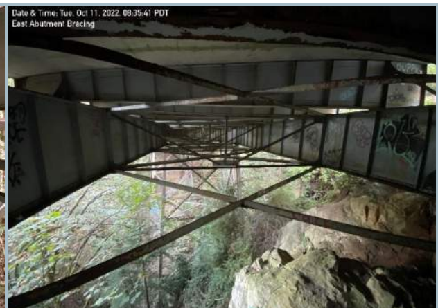
035. Horizontal Cross-Bracing and Intermediate Vertical Lateral Bracing Elements, Typ.
