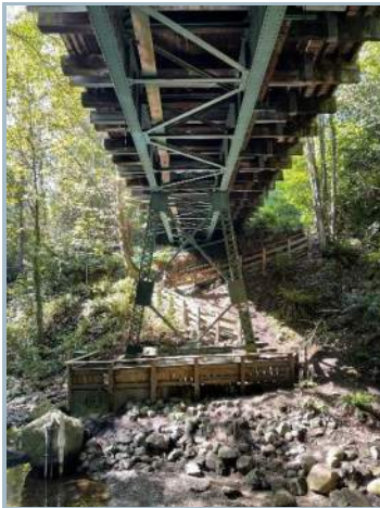
009. West Pier Abutment
