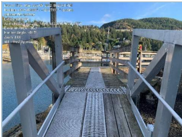
015. Gangway Access Approach to Timber Pier (Note: Skewed Corner Orientation)
