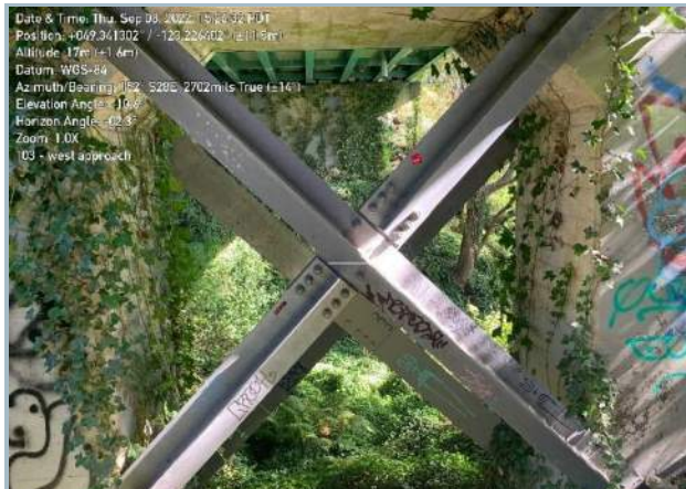
021. Lateral Bracing at West Pier
