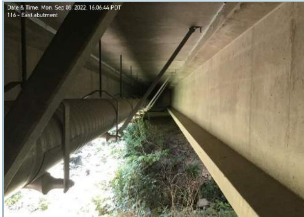
012. Watermain Utility Along North Profile
