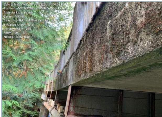
026. South Profile Parapet
