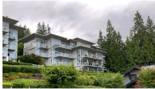
Boulders, West Vancouver
