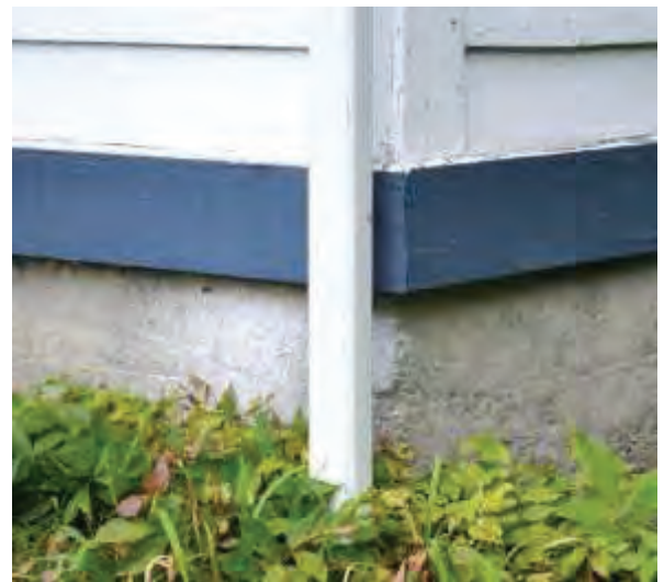
Figure 27: Base plate below siding
