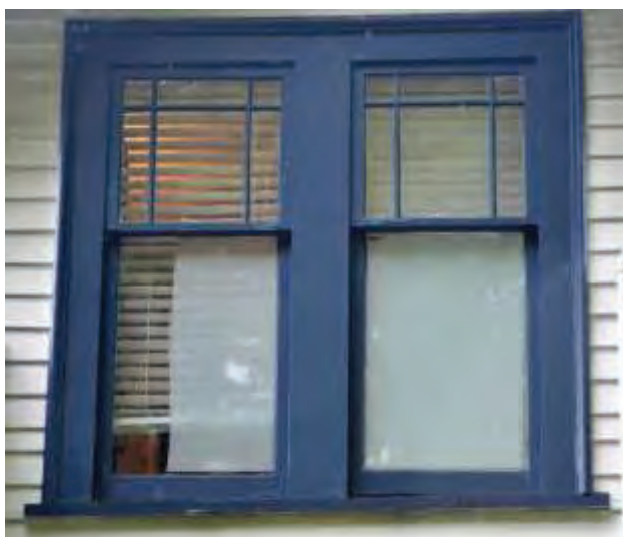
Figure 40: Dormer pair of multi pane double hung windows (WS-4)
