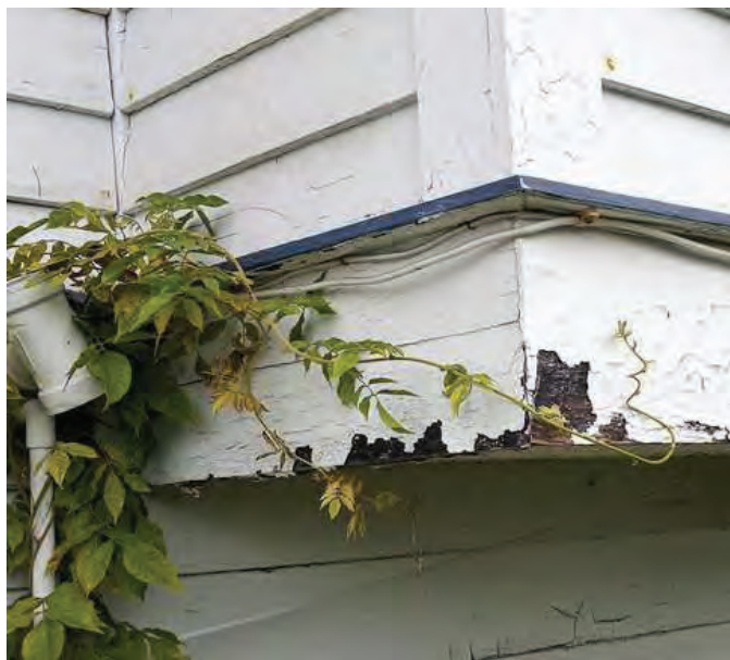
Figure 63: Peeling of siding paint and vegetal invasion
