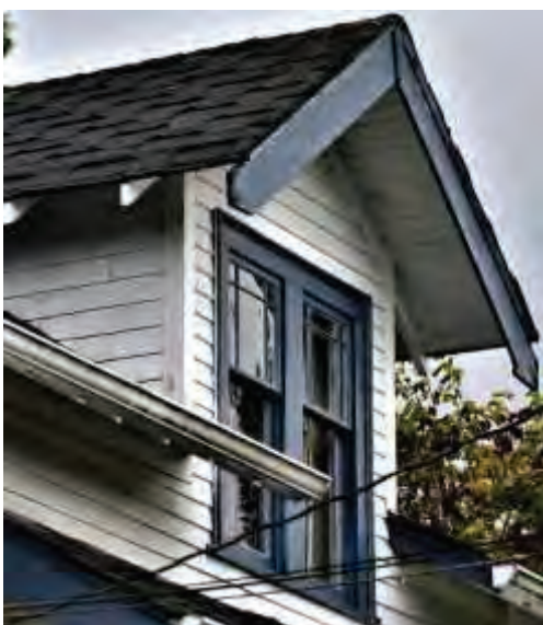
Figure 22: Shingle dormer cheek at south elevation
