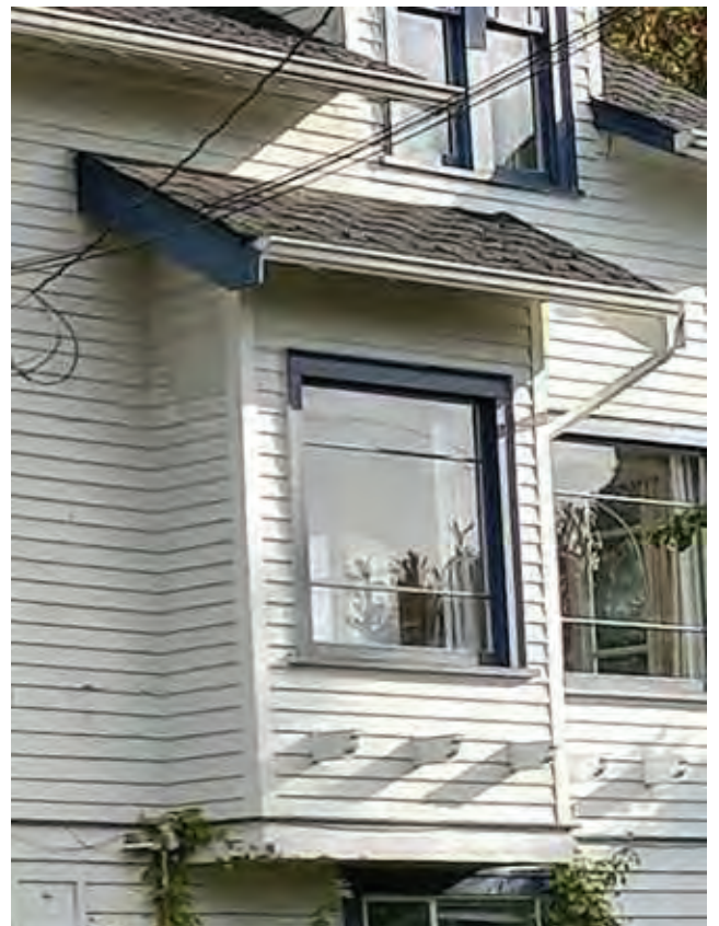
Figure 53: Box window with shed roof (WS-2)
