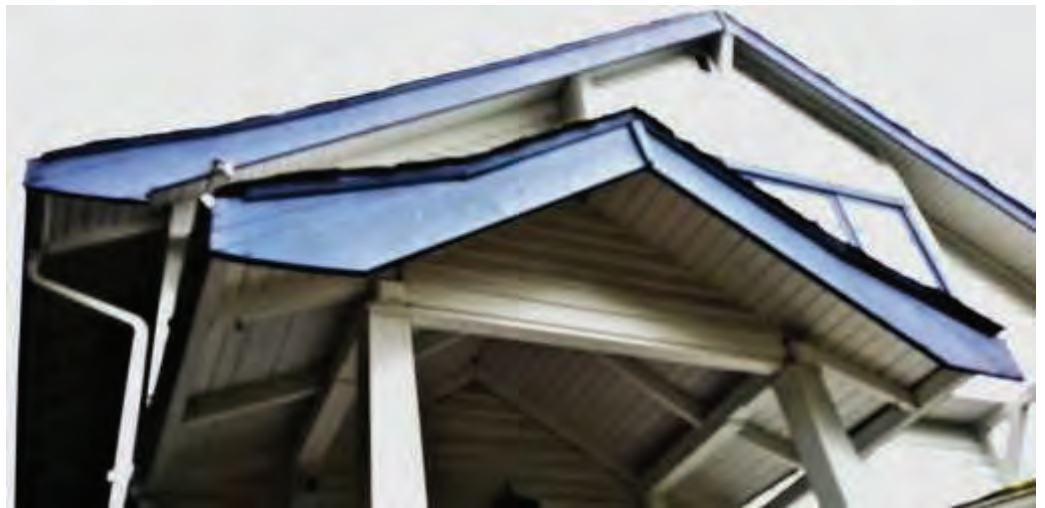
Figure 31: Front porch barge board and overhang
