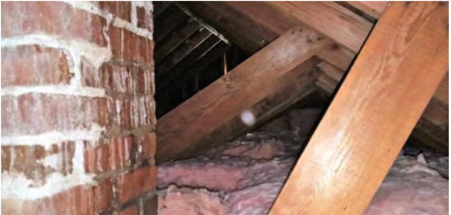
Figure 60: Chimney through attic space, with wooden trusses and bat insulation on above ceiling
