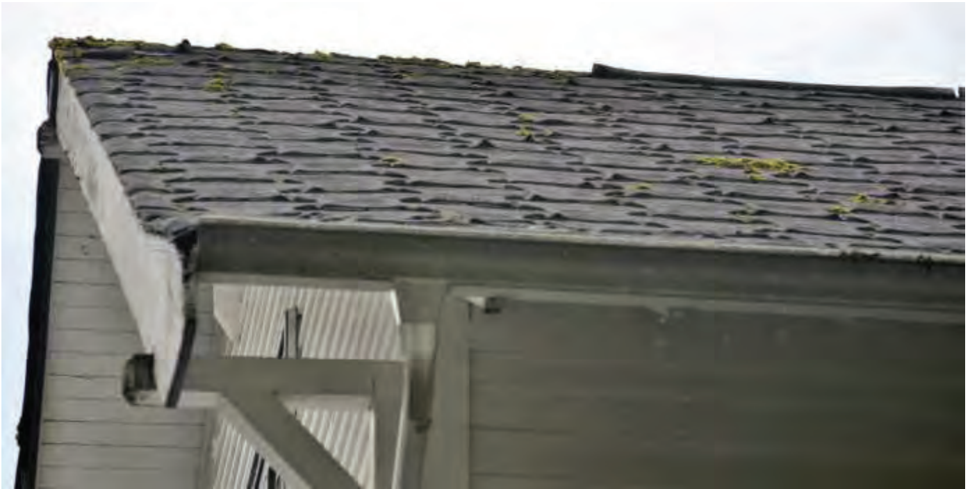
Figure 21: Vintage asphalt roofing with gable end bargeboard and knee-bracket on the left and eavestrough on the right
