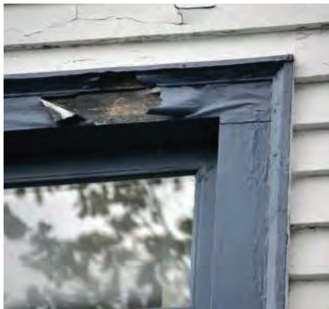
Figure 64: Peeling of window trim paint
