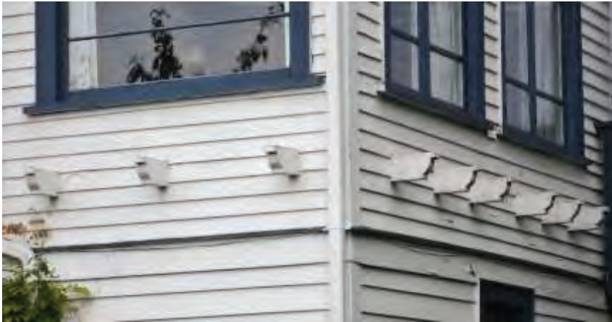
Figure 28: South and east elevation flower box studs
