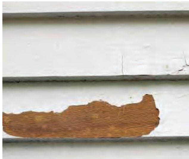
Figure 62: Natural look of siding beneath the white paint
