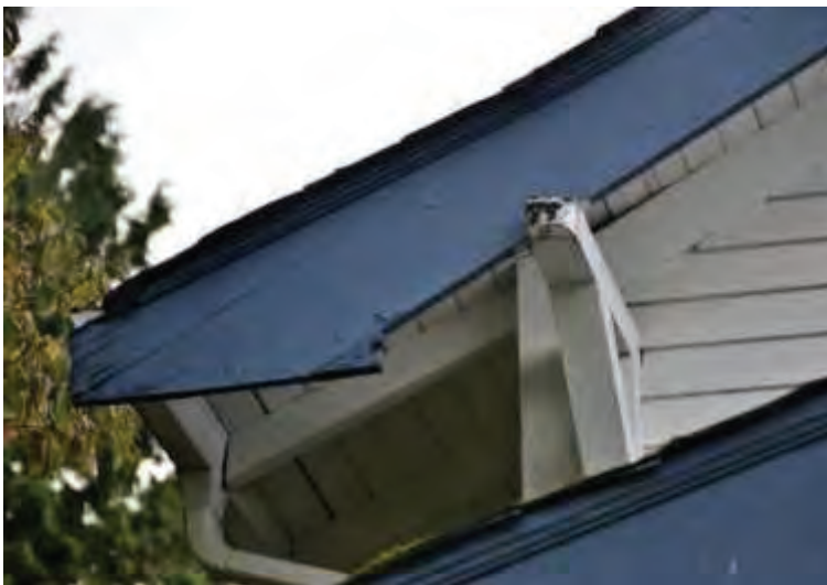
Figure 26: Headboard above siding
