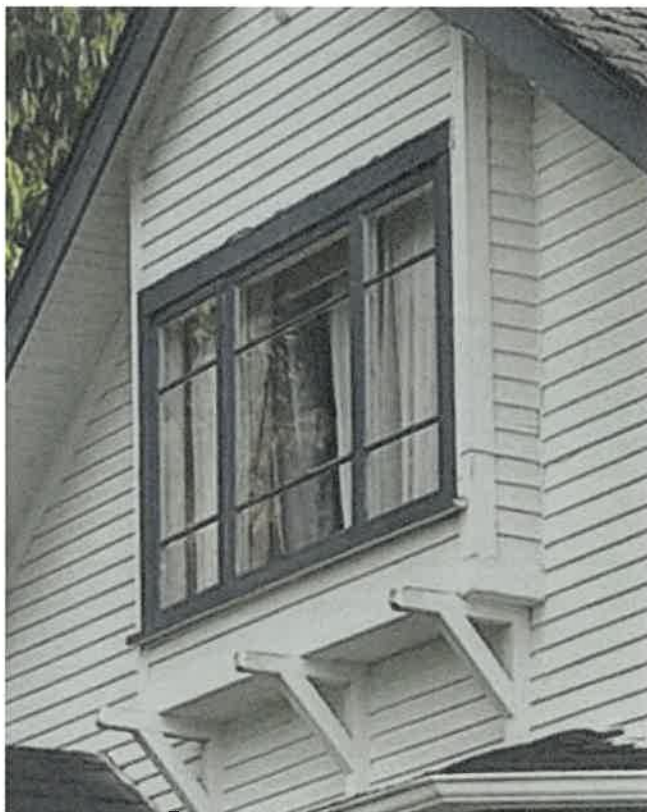
Figure 52: Box window with knee-brackets (WW-2)
