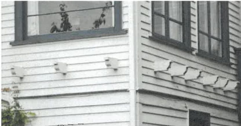
Figure 28: South and east elevation flower box studs
