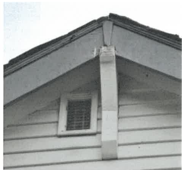
Figure 20: Knee-bracket at gable end's, moulding and key with attic vent
