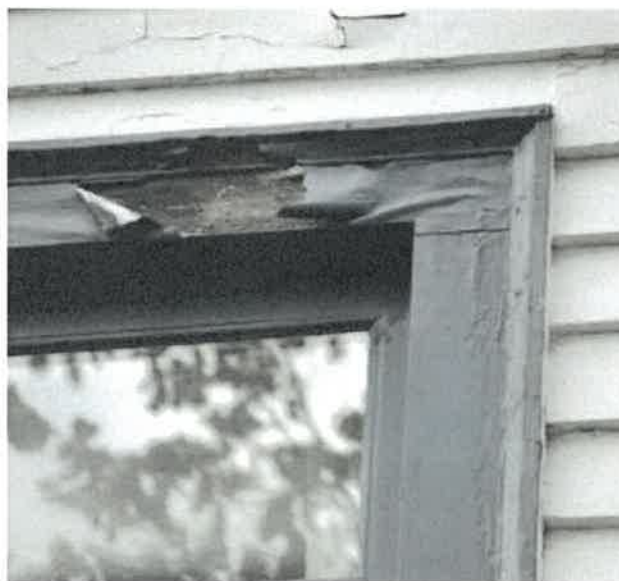
Figure 64: Peeling of window trim paint
