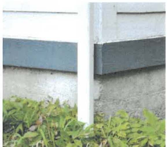
Figure 27: Base plate below siding
