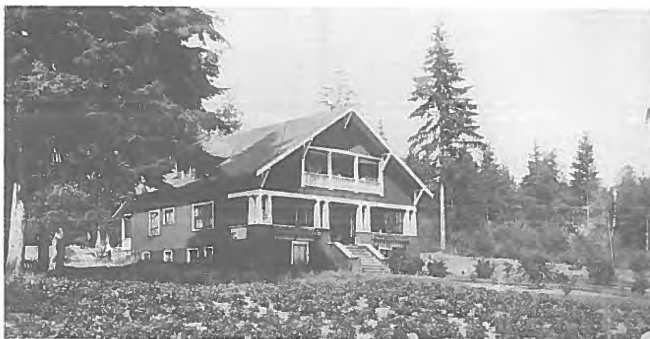
Archival image of the Vinson Residence [source unknown]
