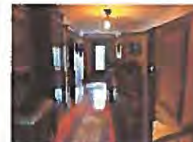
The upstairs vestibule will be retained but modified to accommodate the new bedroom and bathroom layouts
