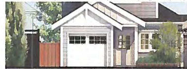
The laneway cottage has its entry from the rear lane. There is a second entry from the street 11
