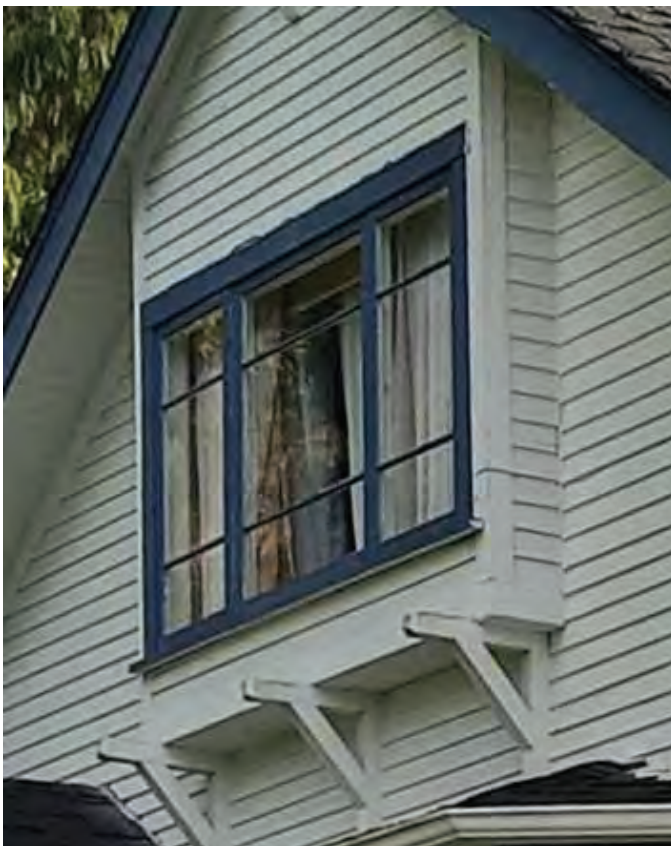
Figure 52: Box window with knee-brackets (WW-2)
