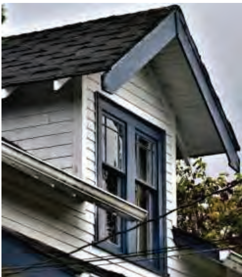
Figure 22: Shingle dormer cheek at south elevation
