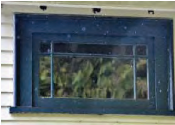
Figure 46: Fixed multi pane window (WN-2)
