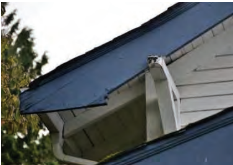
Figure 26: Headboard above siding
