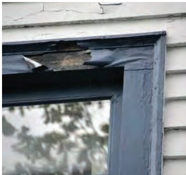
Figure 64: Peeling of window trim paint
