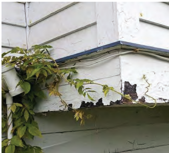
Figure 63: Peeling of siding paint and vegetal invasion
