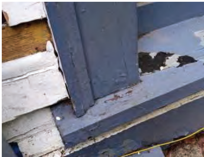
Figure 61: Black trim colour beneath the blue accent paint
