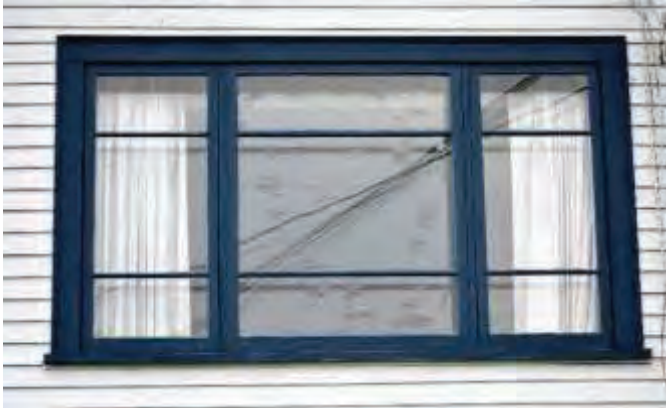
Figure 44: Multi pane fixed with casements on both sides (WS-1)
