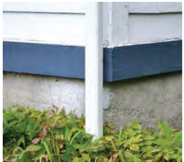
Figure 27: Base plate below siding
