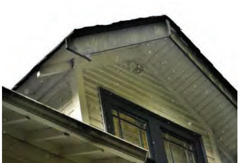
Figure 23: Front of typical dormer with bargeboard, exposed rafter and open soffit
