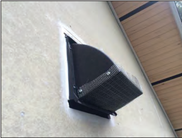
Figure 2. Standard exterior vents. Left: covered with 3mm wire mesh. Right: vent with open flap
