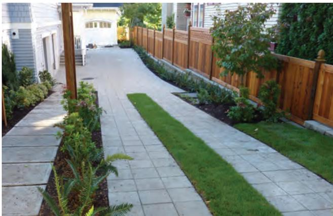
**Fig 2.8:** Where driveways are required, consider alternative paving materials that reduce runoff.
