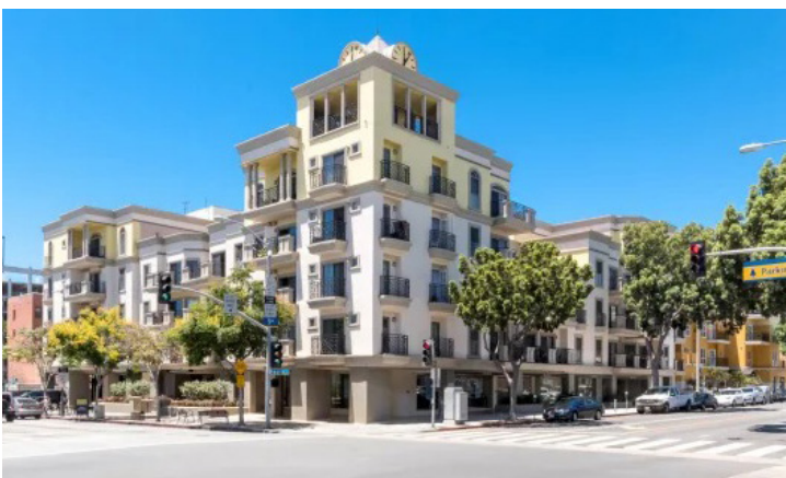
Selectively introducing additional height both within and between buildings can add visual interest and create a more sculpted skyline (Santa Monica) | Source: Equity Apartments
