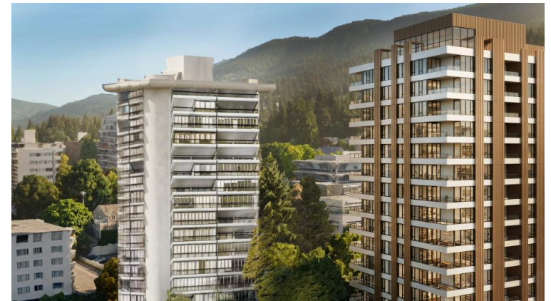
View from the Existing Rental Tower
