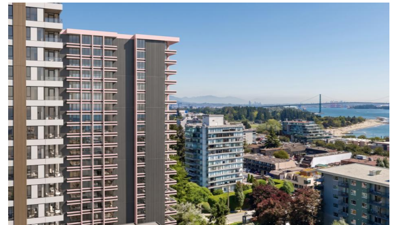
View from Westshore Place Residential Tower
