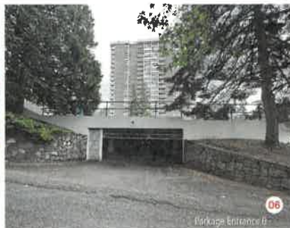
Parking Entrance B
