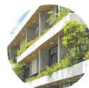
Integrated planters on balconies
