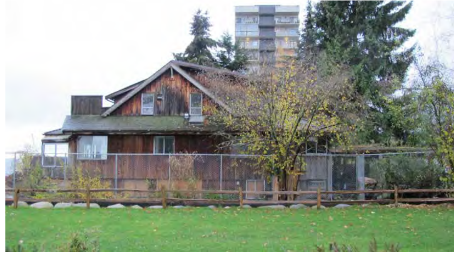
Existing East Elevation. November 2020
