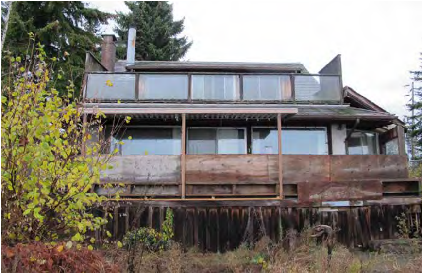
Existing South Elevation. November 2020
