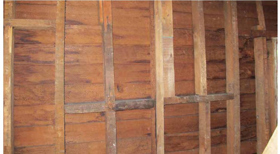
Backside of exterior cladding.
