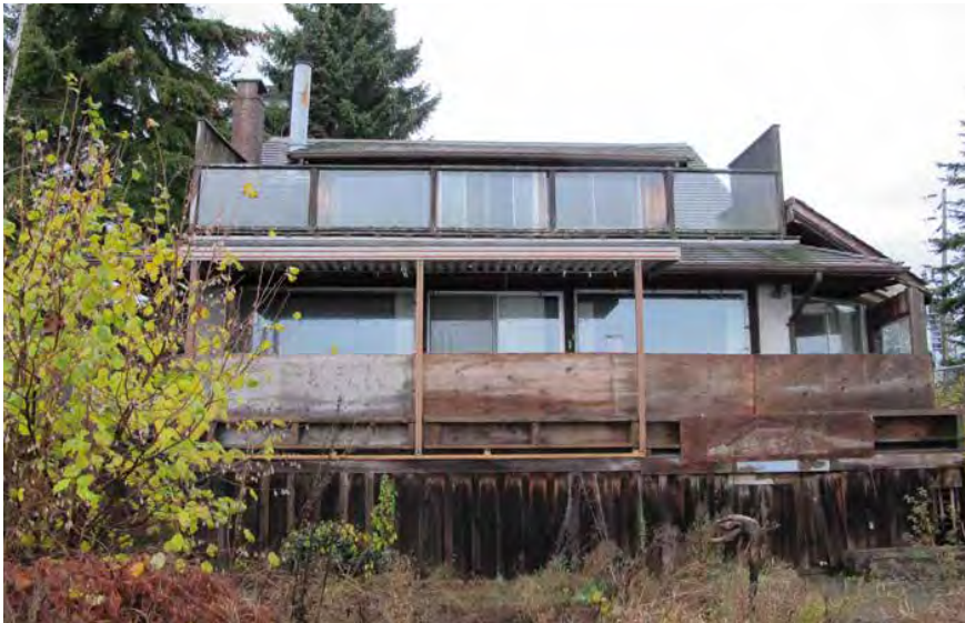
Existing South Elevation. November 2020
