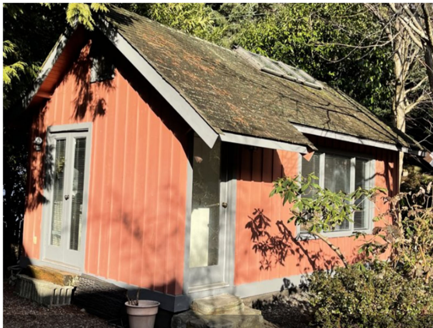
Figure 5 – Photograph of small residence located on the subject site
