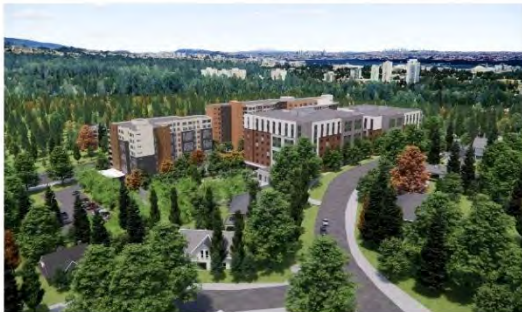
NORTHWEST CORNER View from the north-west corner of the site with the Long Term Care buildings to the right and their secure garden space to the left.
