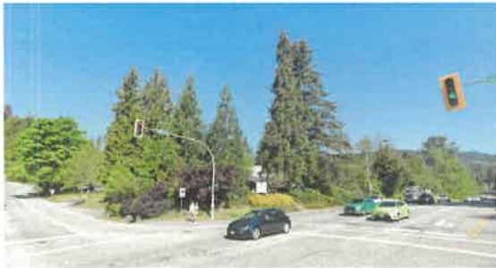
1 Taylor Way at the junction of Inglewood Ave.
