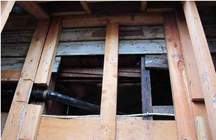
Siding behind later construction, Ground Floor East Side
