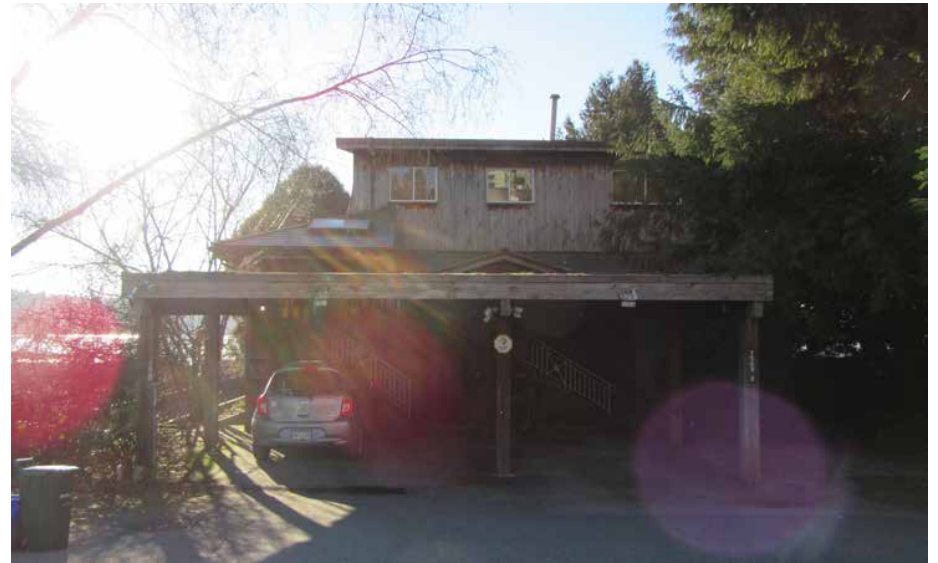
Existing North Elevation. January 2017
