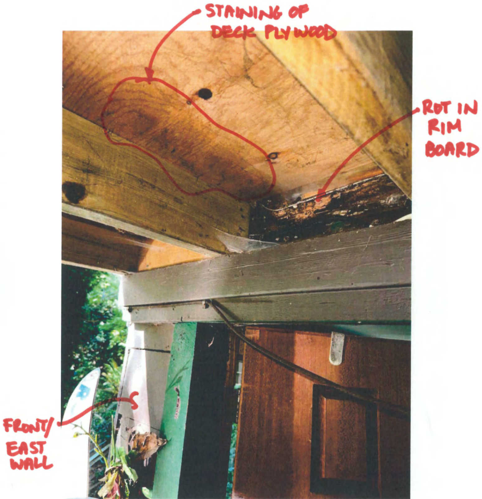
2nd FLOOR DECK & RIM BOARD
