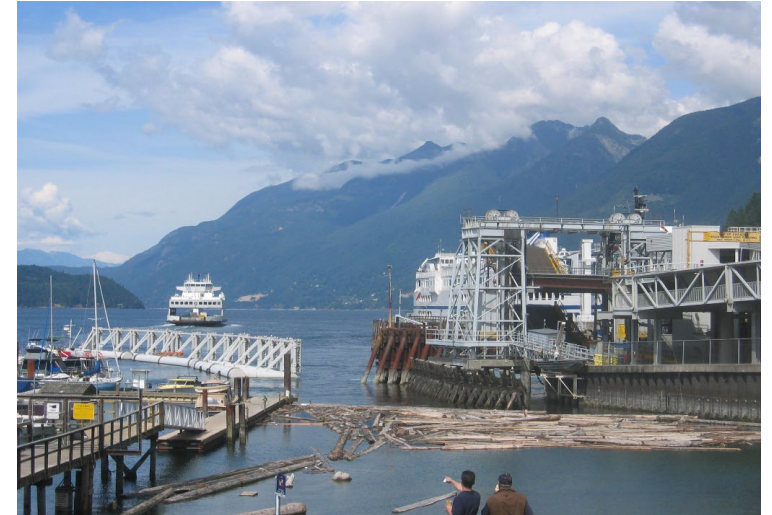
Wikipedia.org – Horseshoe Bay Ferry Terminal
