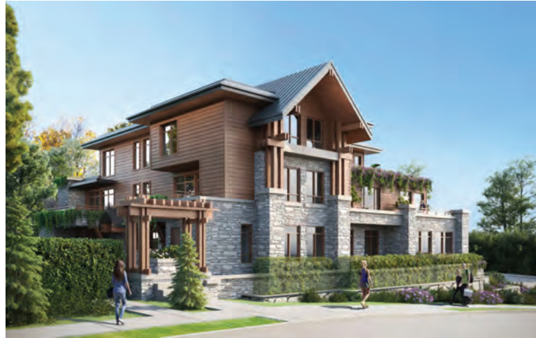
VIEW FROM MARINE DRIVE (SOUTH WEST)
