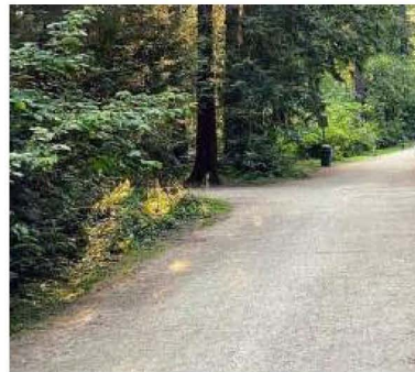
Compacted gravel at rear yard exit walkway
