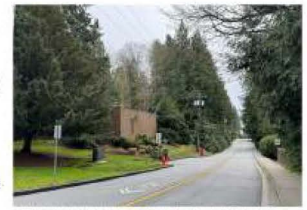
EXISTING UTILITY BUILDING ALONG MARINE DRIVE - VIEW FACING SOUTH
