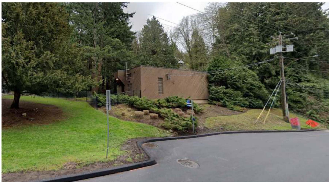
Figure 3: Existing Telus Building at 6085 Marine Drive
