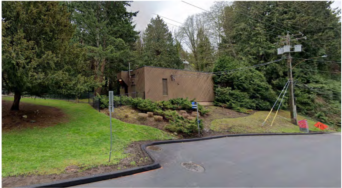
Figure 3: Existing Telus Building at 6085 Marine Drive
