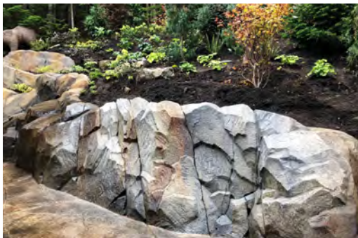
Cast in Place - Shotcrete Feature Wall
