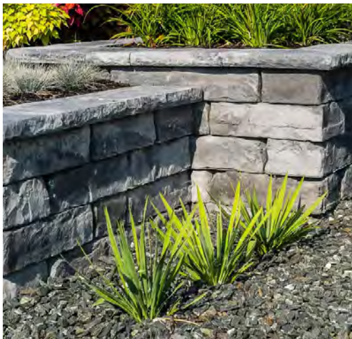
Rosetta Kodah - stone faced retaining wall
