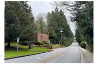
EXISTING UTILITY BUILDING AT 6085 AND 6093 MARINE DRIVE - VIEW EAST, SOUTH
