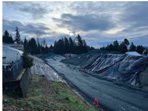
Image 4: Removal of unsuitable sub-grade materials
