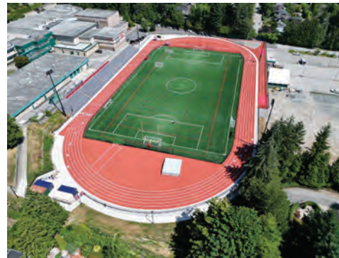
Image 16: Completed track and field
