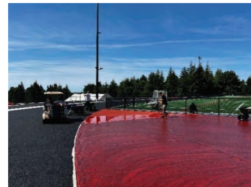
Image 14: Rubber running track installation
