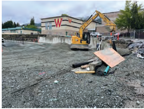
Image 7: Installation of NE retaining wall
