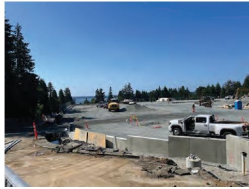
Image 8: Installation of NE retaining wall
