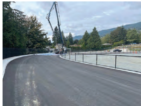
Image 10: Asphalt base for running track
