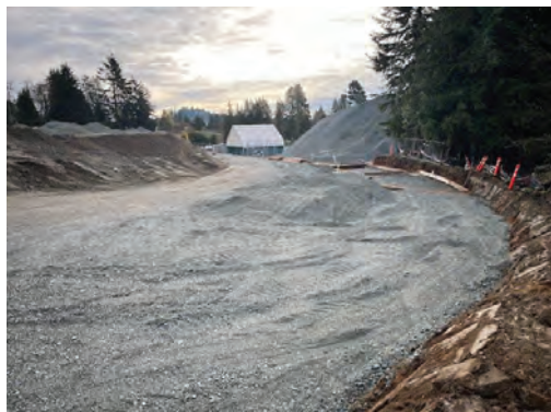
Image 5: New gravel base for running track
