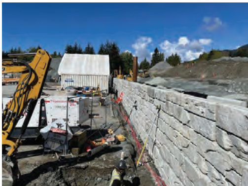
Image 6: Construction of south retaining wall
