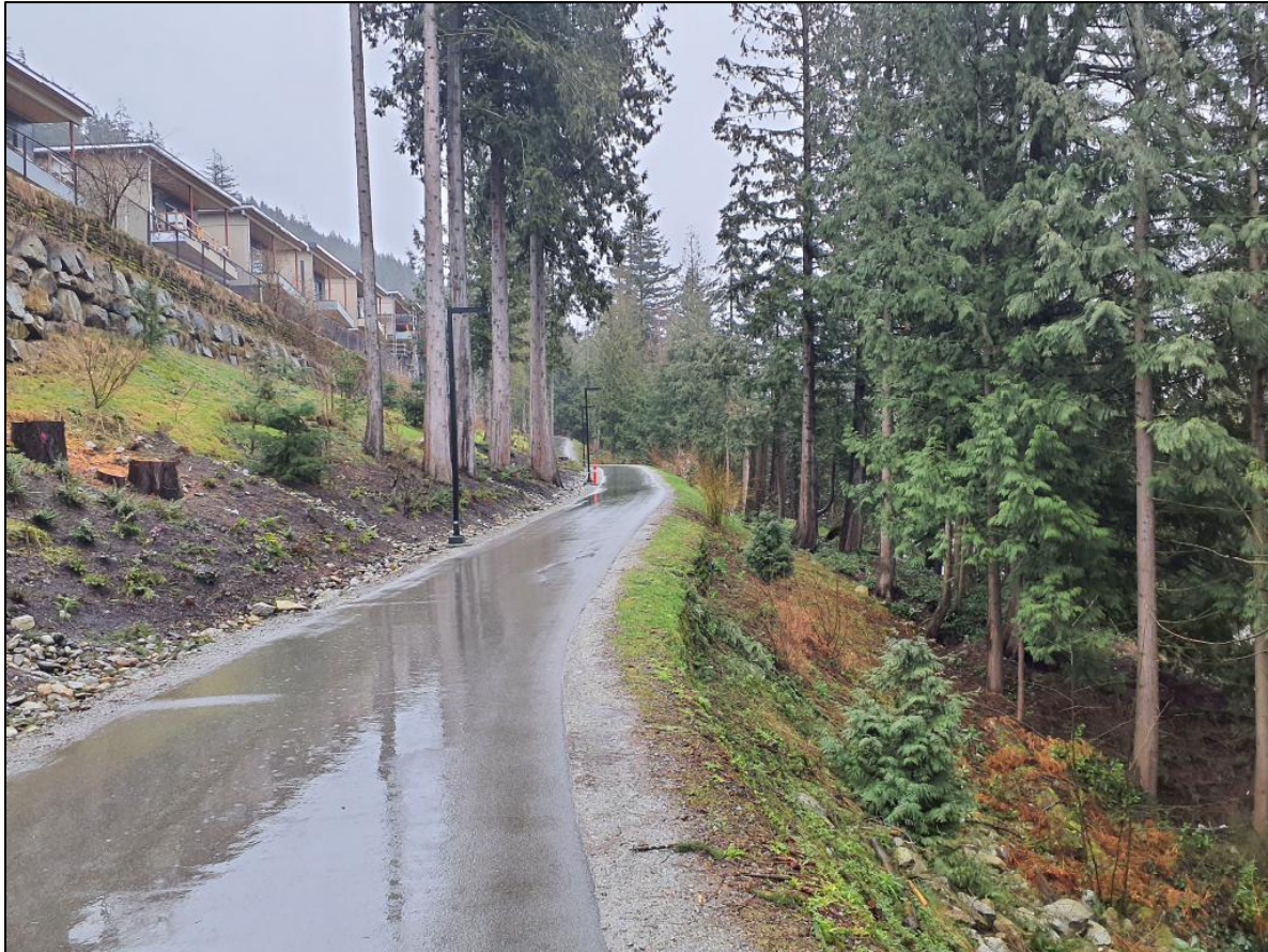
Figure 9. Example of proactive vegetation management and emergency access in Area 6: 1) conifer trees removed or pruned on the high side and deciduous shrubs planted; 2) deadfall removed, trees spaced and pruned on the low side; 3) paved access to the interface area downslope of structures.
